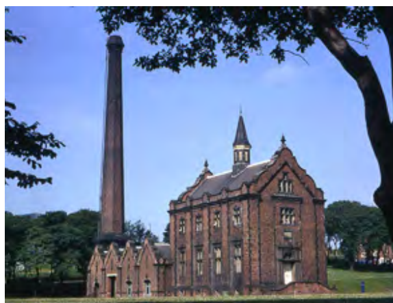
Figure 3. Ryhope Pumping Station Sunderland
