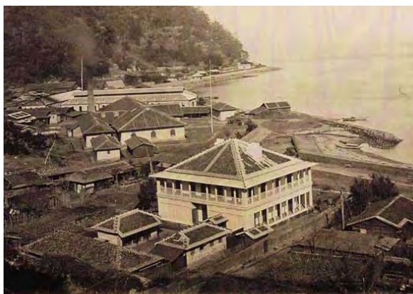
Figure 8. The pioneer factory complex at Shuseikan, next to the Shimadzu summer garden, in Kagoshima, Kyushu, Japan, 1872. Copyright Shuseikan Museum
