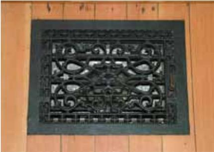
Functional elements, such as radiators and decorative grilles, can contribute to the overall heritage character of a place. Opportunities to retain these features when upgrading or replacing mechanical systems should be explored. This heating grate is one of many that were retained and repaired for use with a new heating plant when the Dawson City Telegraph office was rehabilitated into housing.
