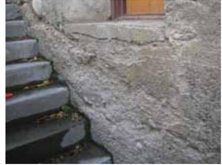
In the early 20<sup>th</sup> century, concrete was still an experimental material. The early designers and fabricators did not have full knowledge about the properties and characteristics of the concrete or its performance in the Canadian environment. Early examples of concrete construction often have inherent problems, are in poor condition and can require considerable conservation work.
