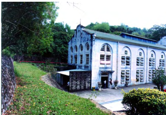
Figure 3. The hydraulic power plant in southern Taiwan
