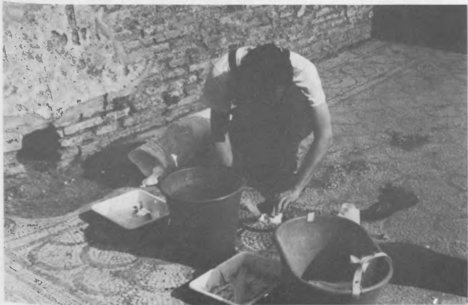
FIGURE 5. Ostia Antica. Injection of Primal AC-33.
