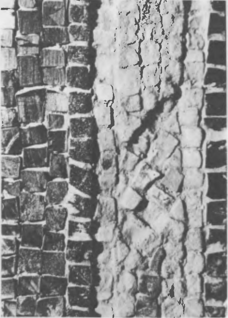
8. Corrosion of white stone, close-up of Apostle N°12.
