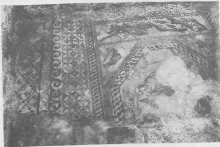
Fig. 1. The mosaic "Achaean" in Ulpia Oescus stained by moisture seepage prior to conservation.
