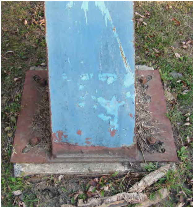
Figure 2 Example of deterioration due to improper maintenance, showing grass projections and scratches from maintenance equipment. Photo: Nathalie Richard, 2012 © CCQ.
