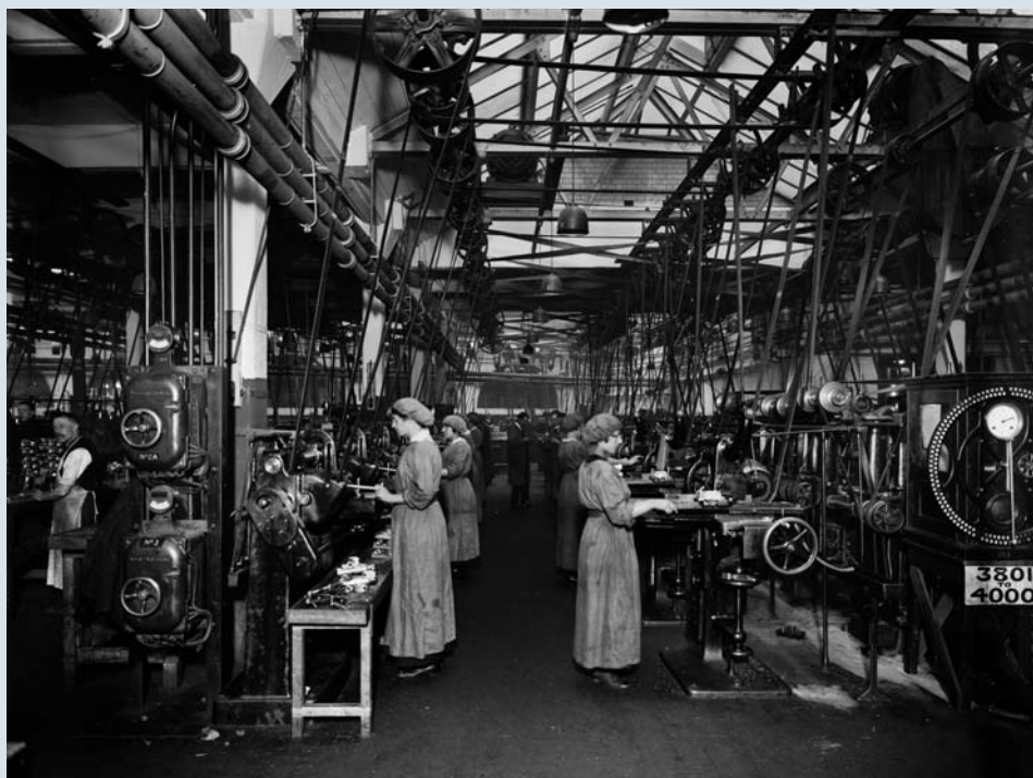
Munitions manufacture on belt-driven machinery in Machine Shop One at the Birmingham Small Arms Company factory in Small Heath. The firm produced rifles, Lewis guns, shells and military vehicles (1917; BL23720/004). Reproduced by permission of English Heritage
