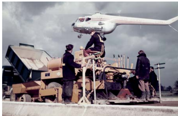
Helicopter and paver on site during construction of the M1 c 1958–59.
