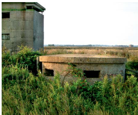
A rare First World War pillbox at East Lane, near Bawdsey on the Suffolk coast. Roger J C Thomas © English Heritage
