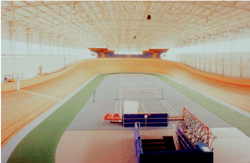
The interior of the seaplane hangar of 1918 at Calshot Activities Centre, which now houses the only indoor banked velodrome in the south of England, tennis courts and other facilities. The hangars at Calshot exemplify better than any other site in Britain the remarkable developments in aero engine and aircraft technology in this period. Mike Williams © English Heritage
