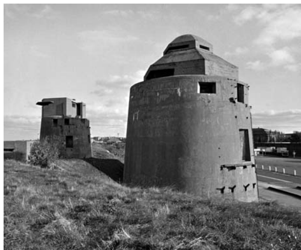
Surviving First World War 4.7-inch gun towers at Centre Bastion, Sheerness, Kent at the mouth of the River Medway. © English Heritage
