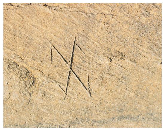
5. Where dressed stone surfaces are not excessively eroded, they may be highly informative. Here the original mason's short diagonal chisel marks are still clearly visible, as is the mark by which the mason identified the stone as his own work. A study of the location of masons' marks within a building can be of help in determining the phases by which it was built, and they may be of use in identifying the movements of masons between building projects.
