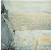
20. Large blocks of stone were a valued building material, and were frequently reused once they had lost their original function. Here part of an early cross slab has been adapted as a lintel in a thirteenth-century stair well. It is important to look out for such stones, though they should only be removed if there are good conservation reasons for doing so.
