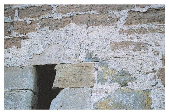
23. Harling tends to survive only in a very fragmentary condition. It is found more often still attached to the rough surfaces of rubble than to smoothly finished ashlar, though in this view it clearly extended across both rubble and ashlar. The coating was sometimes thinner on smoothly dressed stone.
