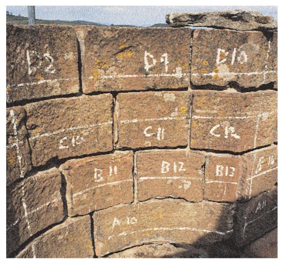
10. Here an ashlar wall-head parapet, which had to be partly dismantled and rebuilt, has had a grid painted across the stones to allow precise re-assembly. Each of the individual stones was also numbered according to its place in the course of which it formed a part. The water-based paint was washed off on completion of the work.
