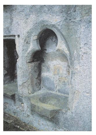
25. Wall plaster does not survive well once a monument has lost its roofs. Where it does remain in more sheltered corners, however, it is clear that it might extend not just across the flat walls but also across the moulded details of any features that were set within the walls.
