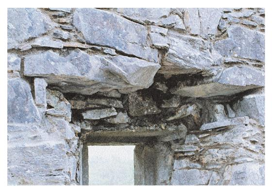
12. The loss of lintels over wall openings can leave the masonry above in an apparently precarious state. However, where the individual stones are of relatively large size, and are deeply bedded in the wall core, the masonry may be less unstable than first seems. Each case has to be individually assessed, but the aim should be to do as little as is consistent with achieving stability.
