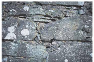
6. The character of rubble masonry varies greatly, according to local traditions, relative date, and the quality of stone available. Where large irregularly-shaped blocks were the main element, the spaces between might be filled with small pinnings, and great care is required to preserve the precise balance between these elements during consolidation.
