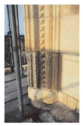
15. Bases tend to take much of the brunt of weathering, and are particularly prone to frost damage. In exposed conditions it is therefore sometimes impossible to be entirely certain of their intended profile. In this case, when bases that had failed structurally had to be replaced, their profile was simply blocked out.
