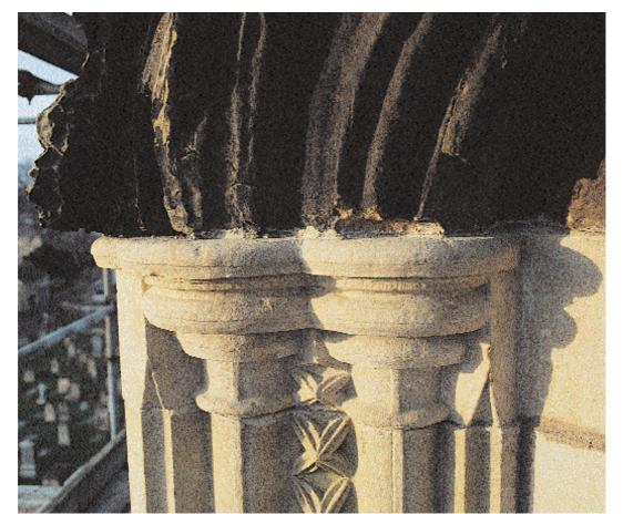
14. In this case, although the engaged angle shafts were so decayed that they were no longer fulfilling their structural role, it was possible to establish the original details from the surviving evidence. Having been carved on the bench, the replacement shafts and caps have been inserted in place and are awaiting final adjustment.
