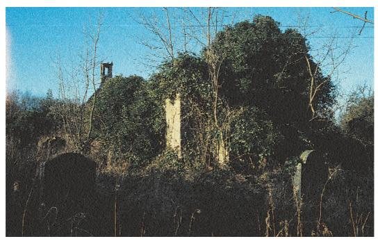
43. In many cases, ivy has taken such a complete hold of a monument that the masonry is almost completely lost to sight. More importantly, however, the ivy will be certainly forcing its way into the joints and core of the stonework, while the constantly increasing weight of the growth may be a major threat to stability.
