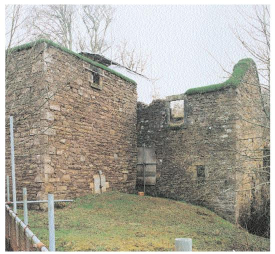
11. In this view the wall-heads of a nineteenth-century mill building have been experimentally protected with turf strips, although this is a technique that is probably more generally appropriate for less complete structures.
