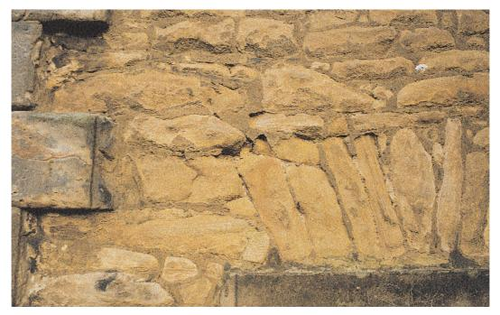
22. Hard cement pointing can exacerbate masonry decay. Here some of the relatively modern cement pointing has been left proud of the adjacent stones as they have eroded. In other areas it can be seen that the original lime mortar survives within the narrow underlying joints where the cement has fallen away.
