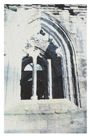
13. The loss of some of the form pieces of this window tracery, and the friable condition of the stone itself, left parts of the window in an unsafe condition. Non-ferrous metal strips, discreetly set into the glazing chases have provided firm support.
