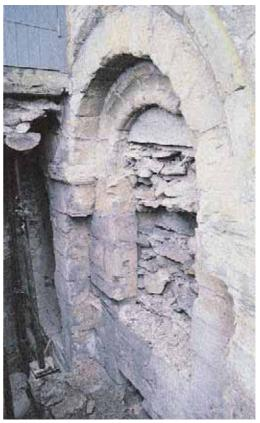
16. This fine Romanesque doorway had been largely hidden behind an early nineteenth-century forestair that was built in front of it. The problems of damage caused by water running down the stair against the masonry of the doorway led to a decision to reexpose the doorway so that its conservation needs could be assessed.
