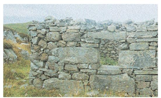
8. Dry-stone construction is common, particularly in 'vernacular' buildings, or in some of the ancillary structures associated with larger monuments. Like rubble masonry in general, it varies according to location, period and availability of materials. Stabilising walls of this kind calls for specialised skills.
