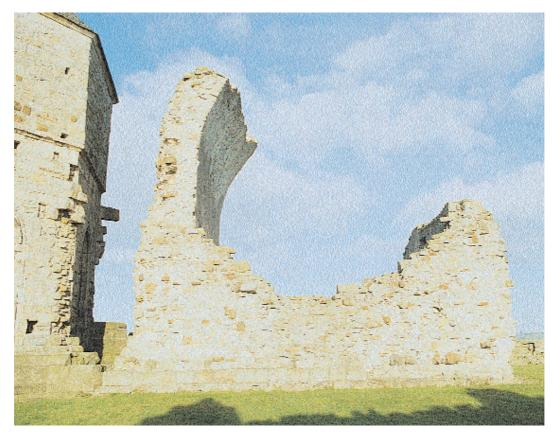
3. Historic masonry may be less precarious than appears on first sight. This apparently gravity-defying section of vault springing shows no signs of further movement.
