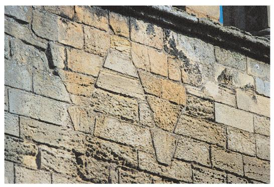
4. Close inspection of masonry may lead to identification of features that were suppressed at later stages of the monument's history. In this case there appear to have been windows alternating with decorative blind arches.
