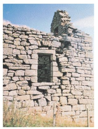
9. Clay was more often used as a bonding material for masonry walls than is generally recognised, even in relatively high-status buildings. Unfortunately, once the wall-head protection is gone, clay is even more easily washed out of the wall core than lime mortar.
