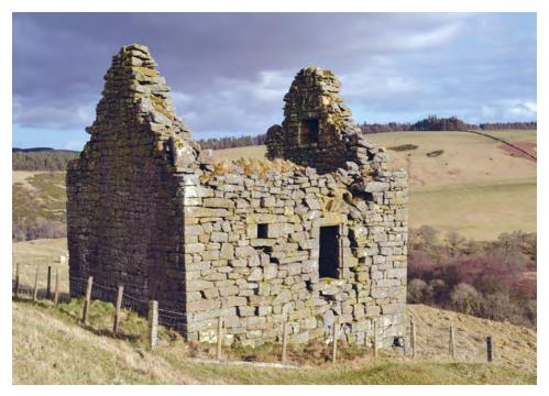
Fig. 3 Mervinslaw Tower in the Scottish Borders dating from c. 1600. Many ruins can appear to be drystone built, however in this case much of the clay mortar has simply been washed out.
