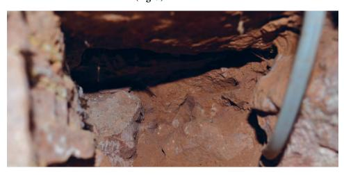
Fig. 5 This opening in a wall has revealed the clay-bonded wall core.
