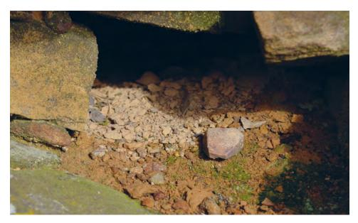
Fig. 4 The remains of clay mortar visible in the wall core at Mervinslaw.
