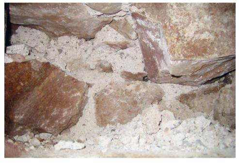
Fig. 7 A lime mortar wall core from the early 19th century, very different in appearance and texture to a clay mortar.
