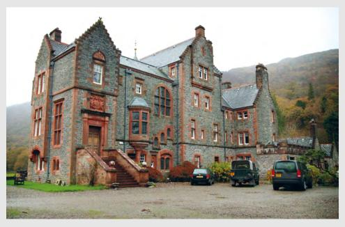
Fig. 1 This 19th century mansion was constructed using clay in the wall core and pointed with lime externally.
