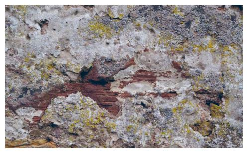
Fig. 10 Remains of a flush point and protective layers of limewash on a wall in the Scottish Borders probably dating from the early 19th century.
