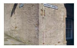
Fig. 2 A clay-bonded wall in Stromness retaining the original lime harl that protects the underlying clay mortar. Masonry walls built using clay often do not differ in external appearance from lime-bonded walls.
