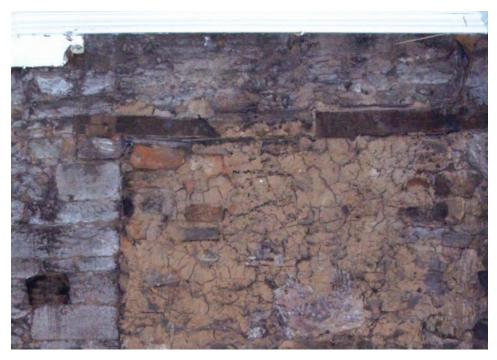
Fig. 8 Interior masonry flush pointed with clay at a 17th century house in Brechin.
