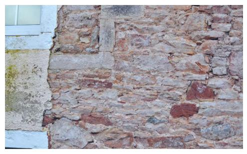
Fig. 9 Dampness necessitated the removal of the cement render from this clay-bonded wall.
