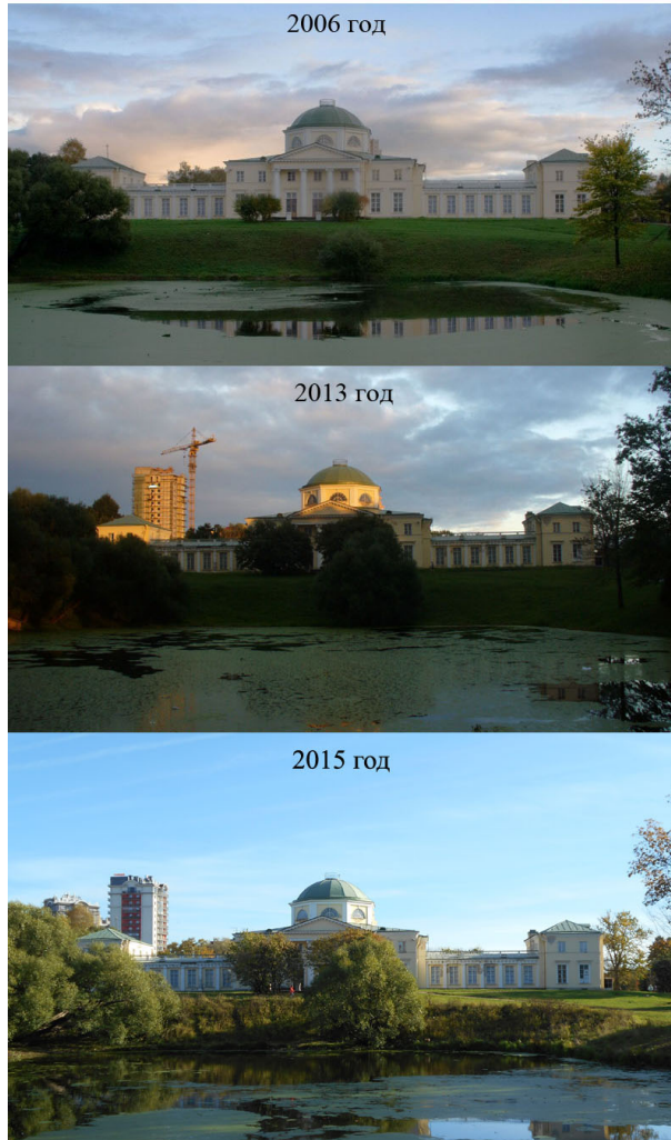
Fig.3- A retrospective of the protected panorama of the Alexandrino Country Estate.
