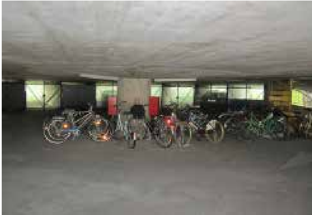
Fig 3: Interior of the Sever car park.
