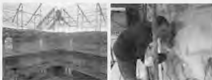
Setting of the scaffolding and cover to protect the walls. A pre-consolidation phase of the ancient marble-plaster, before the winter break.
