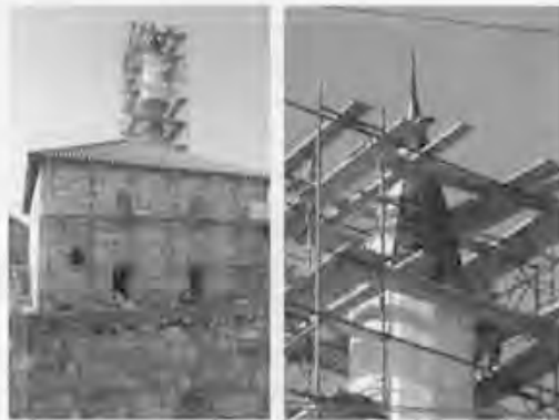
Replacement of wooden elements and installation of new slabs of lead on the cusp of the minaret.
