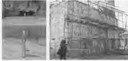
The mechanism of iron designed ad hoc in place of traditional wood stringers, because of conditions of the walls.
