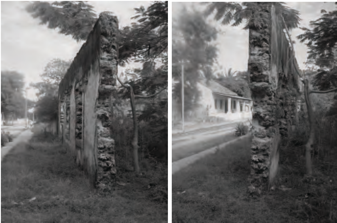
Figure 2.13.: Ruin studied for analysing the behaviour of soluble salts contained in the coral limestone, in Rua Maria Pia [M.B., 2007.].
