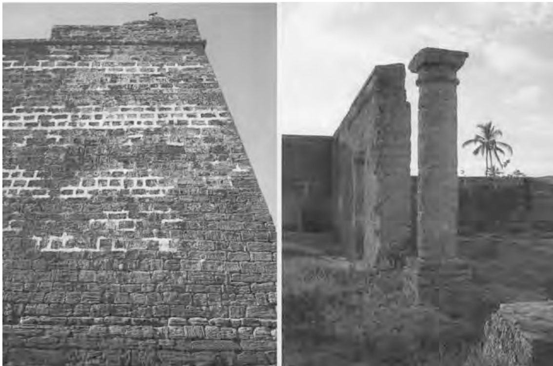
Figure 3.23.: Ilha de Moçambique. The front of a bastion built in limestone blocks of the Tertiary-Quaternary period ( Bioclastic rock ). Column and wall of the ruins of a small house constructed with limestone blocks in a limited stage of diagenesis ( Bioherm rock ) [M.B., 2009.].
