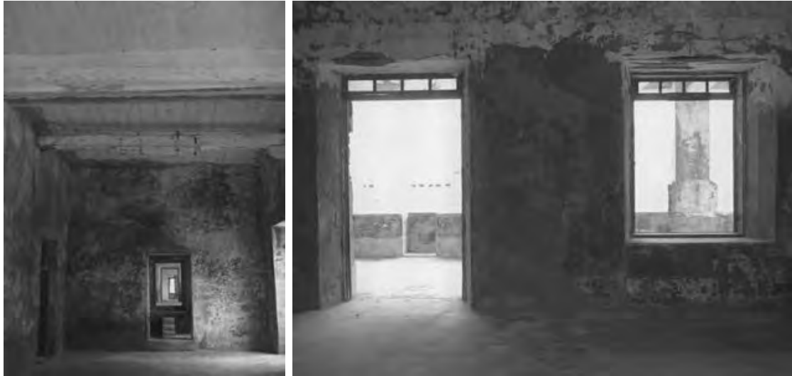
Door and window concrete lintels where iron has broken due to oxidation or corrosion in a normally wet environment and subject to marine aerosol.
