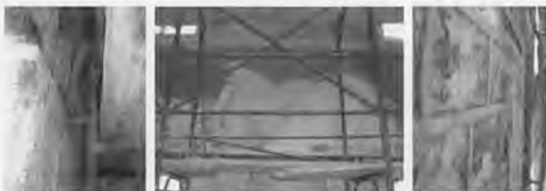
Integration of the missing parts of the "marmorino" plaster in the interior surface of the wall and around the windows at the second order.
