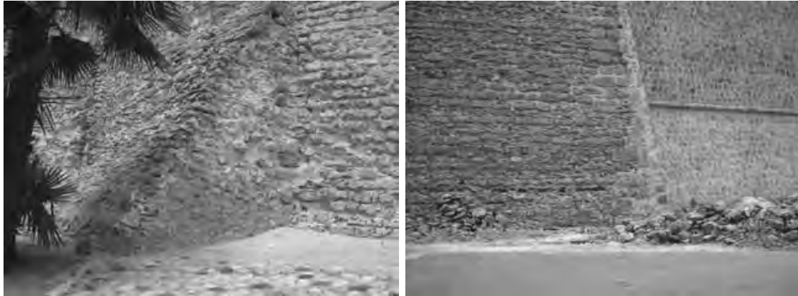
Figure 4.3.: The disruptive effect of salt crystals in the buttress on the side of the Archaeological Museum entrance; the unfinished cladding of the Southwest bastion [M.B., 2006].
