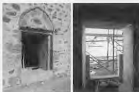
Remaking of the frames of the windows in the same way of the traditional practice.
