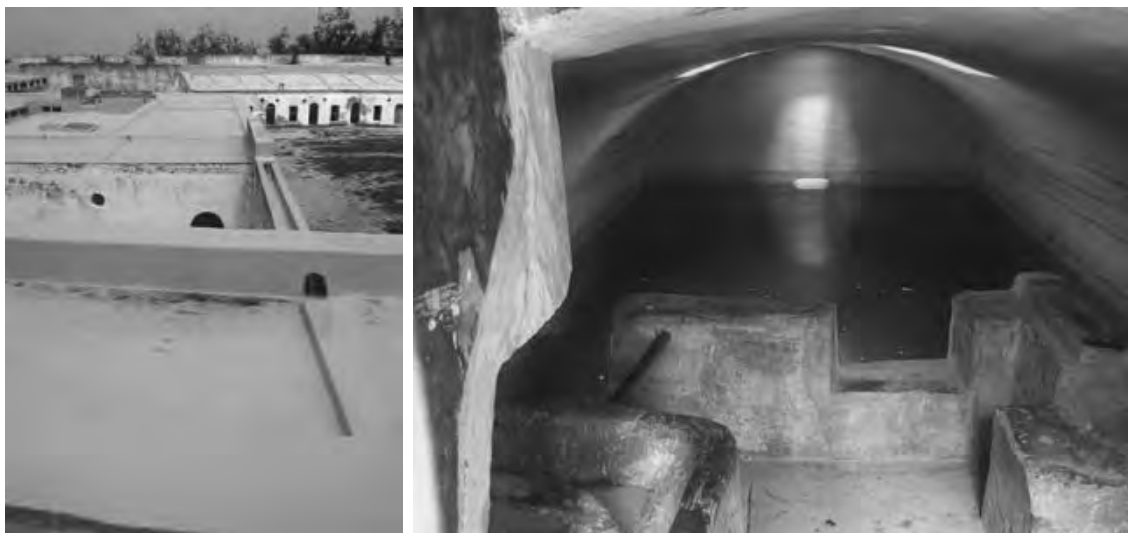
Figure 3.32.: The system for collecting rainwater in the Fortress São Sebastião [M.B., 2009].
