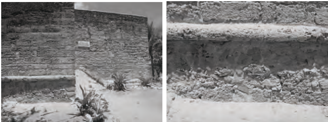
Figure 2.14.: Fortim de São José. Grouting tests after two years from work [M.B., 2007.].
