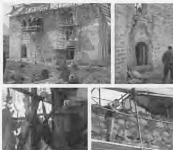
The consolidation operations by injection of lime and replacement of chestnut beams in the walls.
