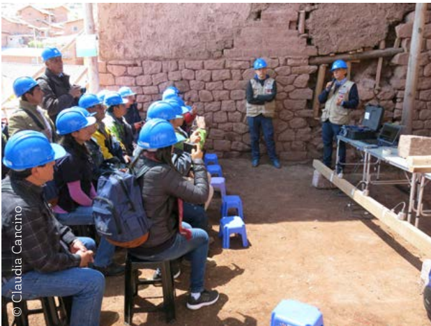
Fig.3 : Non-destructive testing demonstration at Kuñotambo
