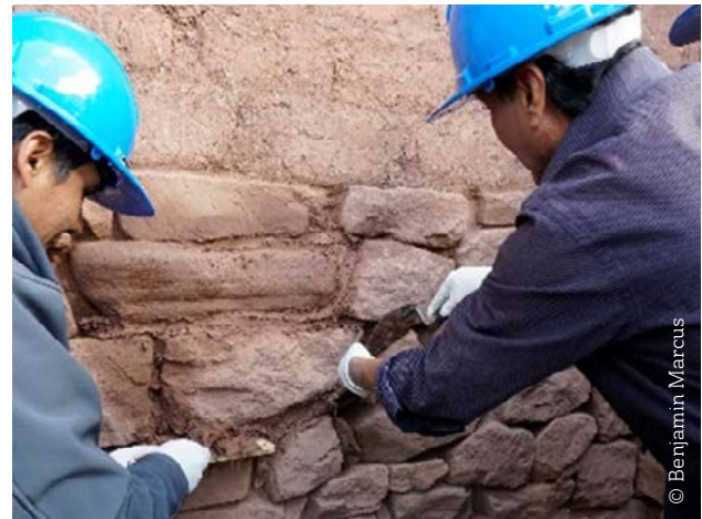
Fig.4 : Workshop Participants repointing a section of masonry wall
