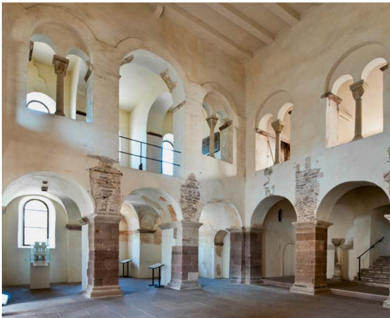
5 Corvey, Church of SS Stephen and Vitus, westwork, west and north walls of the quadrum (873–885)
