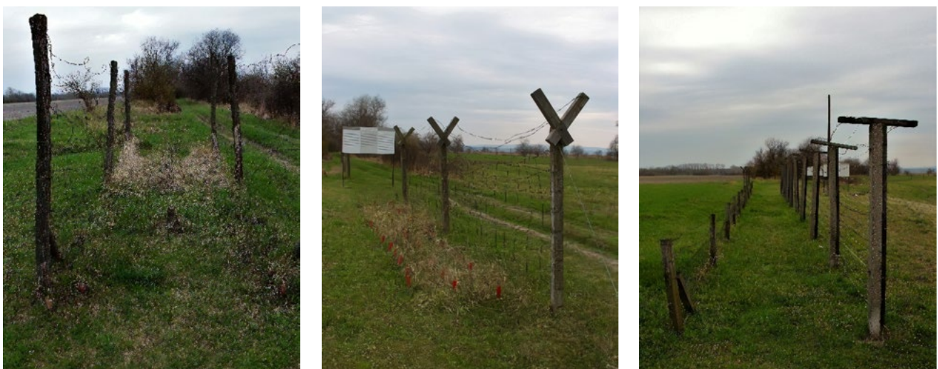
Figs. 16–18: Authentic reconstruction of the three different periods of the technical barrier at Hegykő, at its original location
