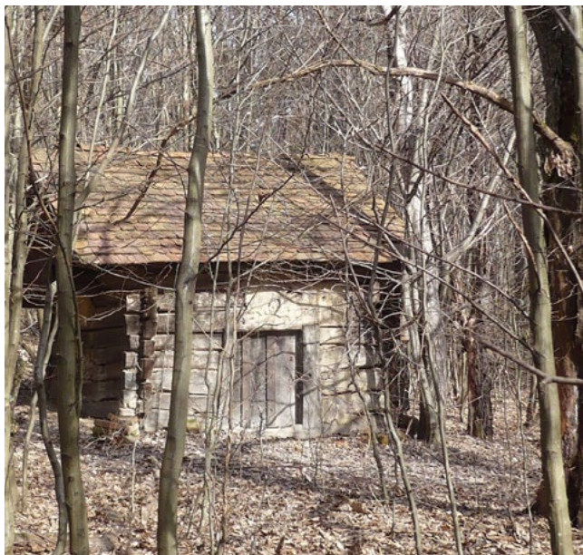
Fig. 32: Forest house near Bajánsenye built 1833
