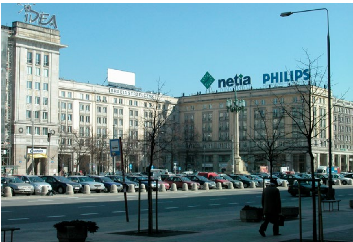
Fig. 2: Marszałkowska Residential District (MDM), Warsaw, south-eastern corner of Plac Konstytucji, Zygmunt Stepiński, Jan Knothe, Józef Sigalin and Stanisław Jankowski, 1949–1952
