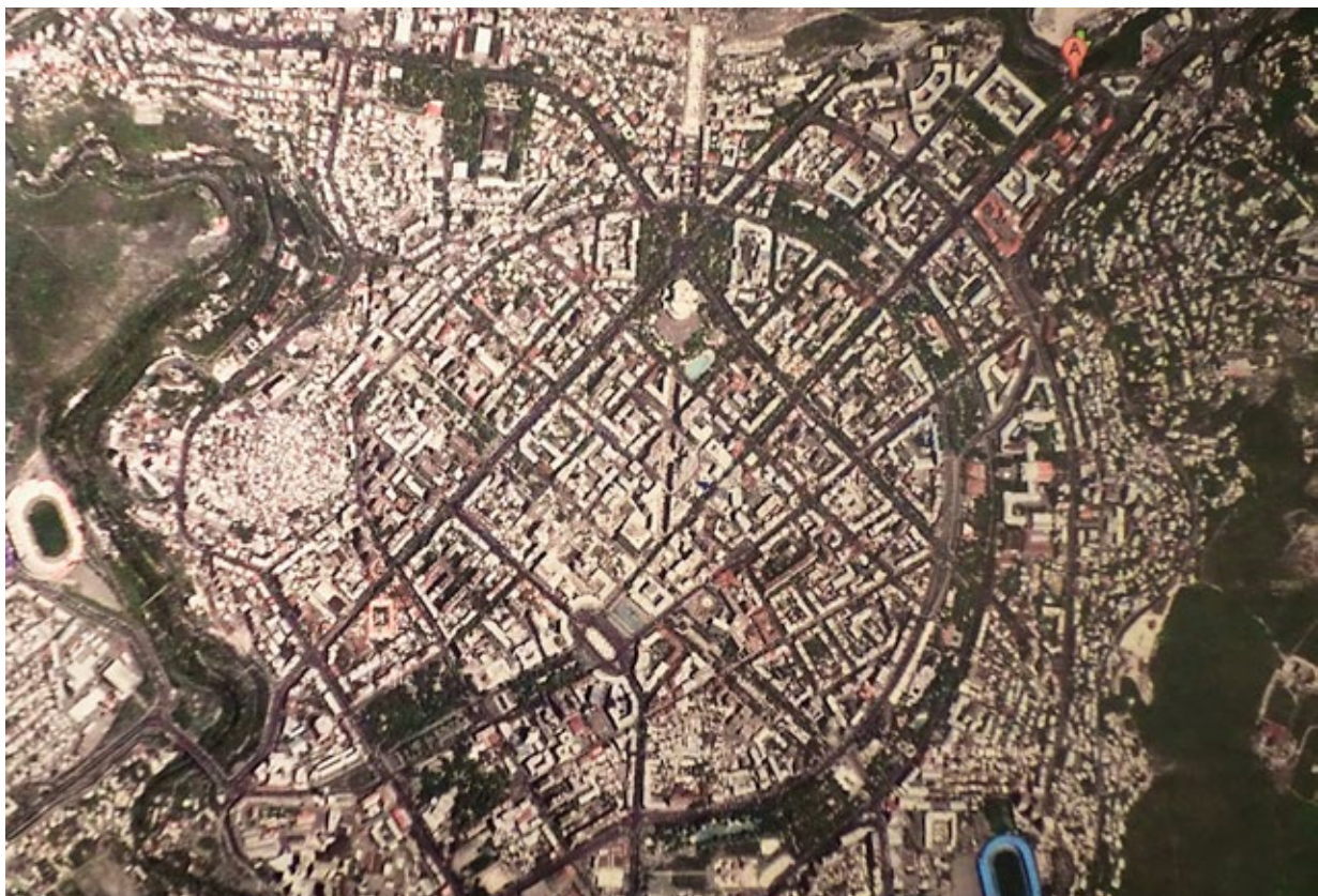
Fig. 7a: Central planning ensemble of Yerevan, the capital of Armenia, aerial view, master plan by A. Tamanyan, 1924
