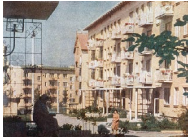
Fig. 10: Nathan Osterman, Sergei Liashchenko and Gueorgui Pavlov, Novye Cheryomushki housing scheme , Moscow, 1956
