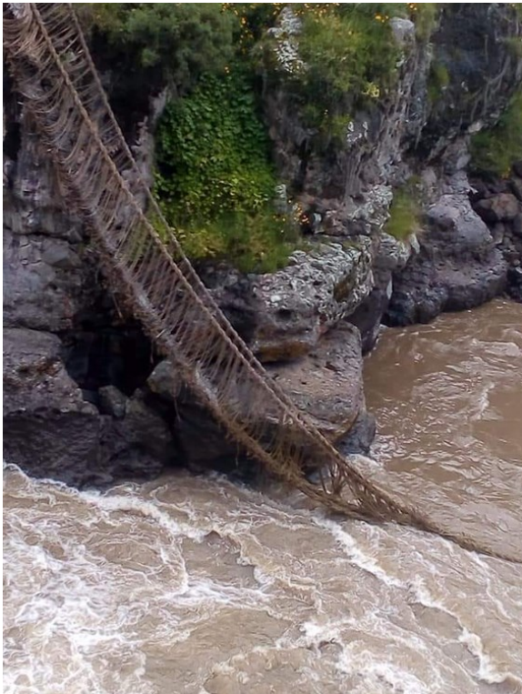
Image 3. "Bridge of the Inca empire in Peru fell due to lack of maintenance because of the pandemic" © Ambito, 2021
