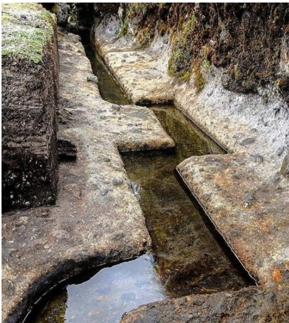
Image 4. Zigzag bends and right angles were used in order to slow down the water velocity © Luis León Pizarro. Travelers Peru - Huaral: Facebook Group 30.01.2012
