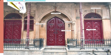
Below: Architectural features of a Haveli
