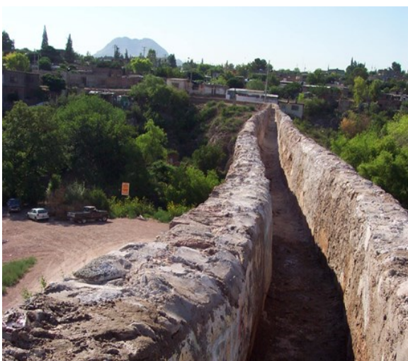
Image 8. Chihuahua Aqueduct, Camino Real Tierra Adentro, México © Cecilia Calderón-Puente
