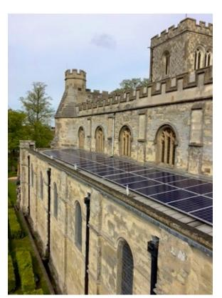
Figure 1. Photovoltaic panels on south aisle of Dunstable Priory © Diocese of St Albans and Dunstable PCC
