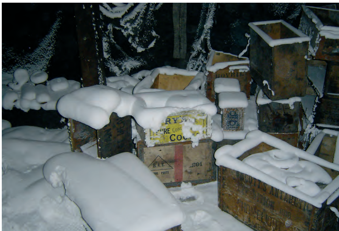
Snow accumulation in the interior of Discovery Hut, August 2007. Photo: Roberta Farrell.
