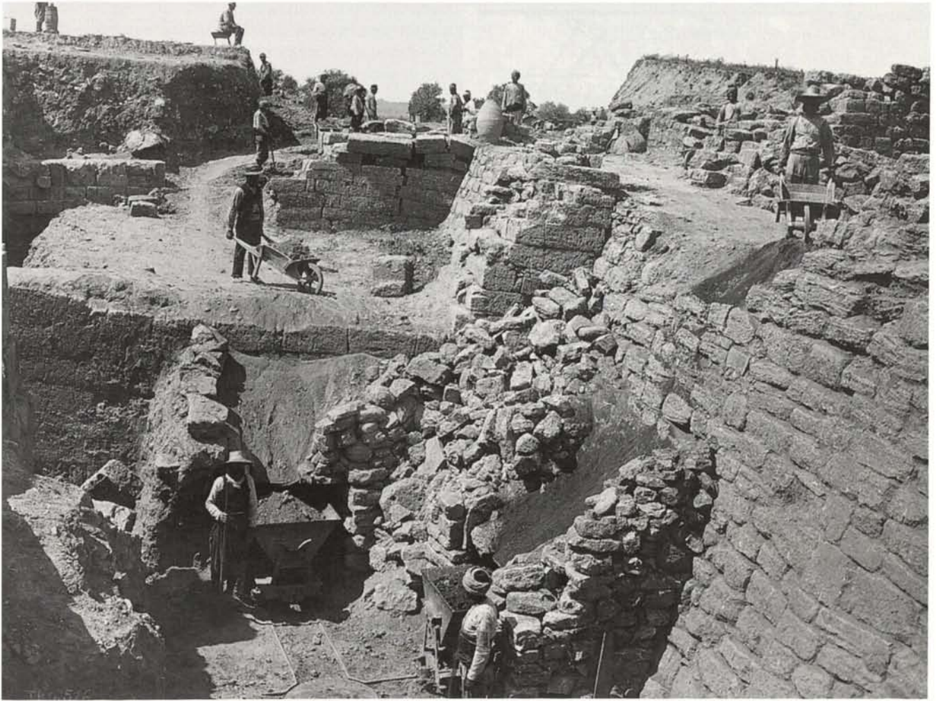
Fig. 1. Troy 1894. Excavation of the fortification wall of the citadel of Troy VI by Wilhelm Dörpfeld in 1894
