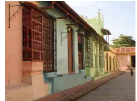
Facades, 18th and 19th centuries in wattle and daub © OHC Camagüey
