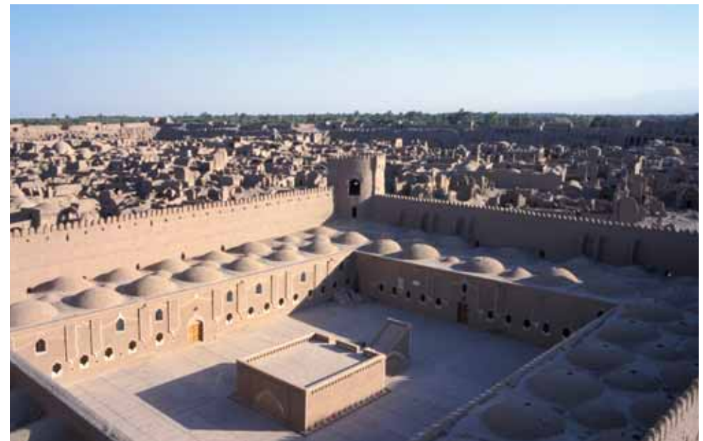
Stable, Citadel of Bam, before its destruction in 2003 © Hubert Guillaud, CRAterre
