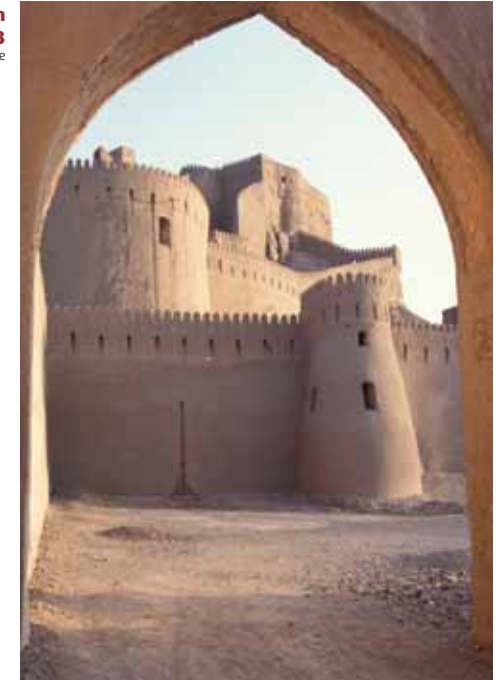
Citadel of Bam before its destruction during an earthquake in 2003 © Hubert Guillaud, CRAterre
