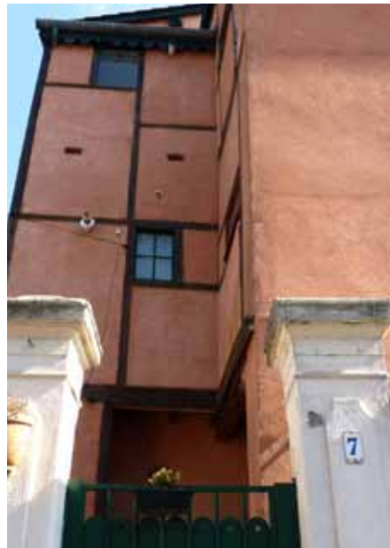
Saint Just quarter, wattle and daub constructions, Saint Fiacre street © Sébastien Moriset, CRAterre
