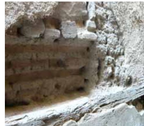
Detail of degraded plaster and of the earth bricks showing underneath
