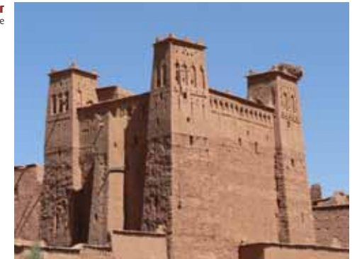
One of the fortified houses of the Ksar © Sébastien Moriset, CRAterre
