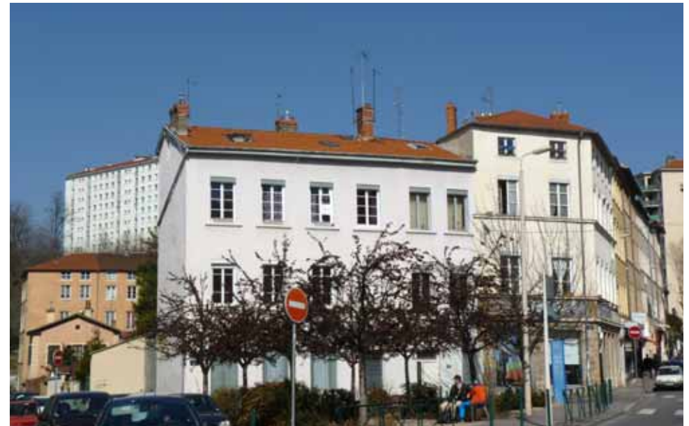
Lyons, Saint Just quarter, rammed earth building at the intersection of Benoist Mary street and 4 colonnes street © Sébastien Moriset, CRAterre
