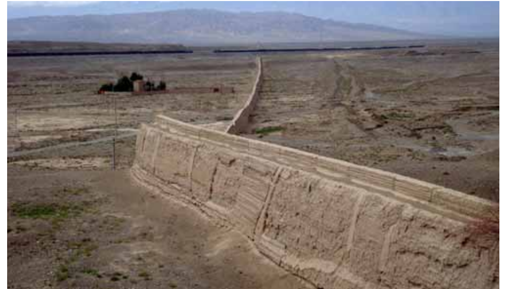
Portions of the Great Wall built with earth
