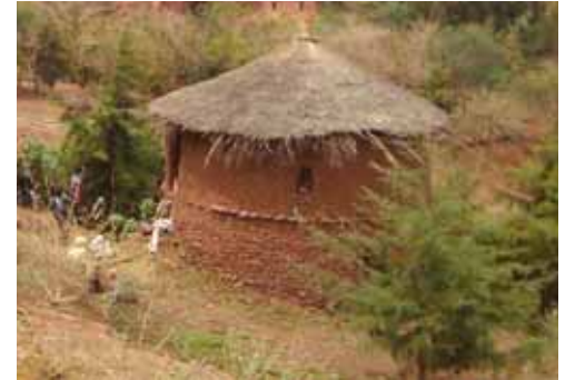
Houses around the famous rock-hewn churches are built of stone walls made with earthen mortars and plasters © Ishanlosen Odiaua
