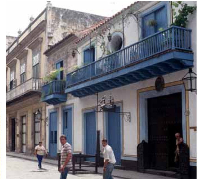
Colonial house built in stone and rammed earth © Wilfredo Carazas-Aedo, CRAterre
