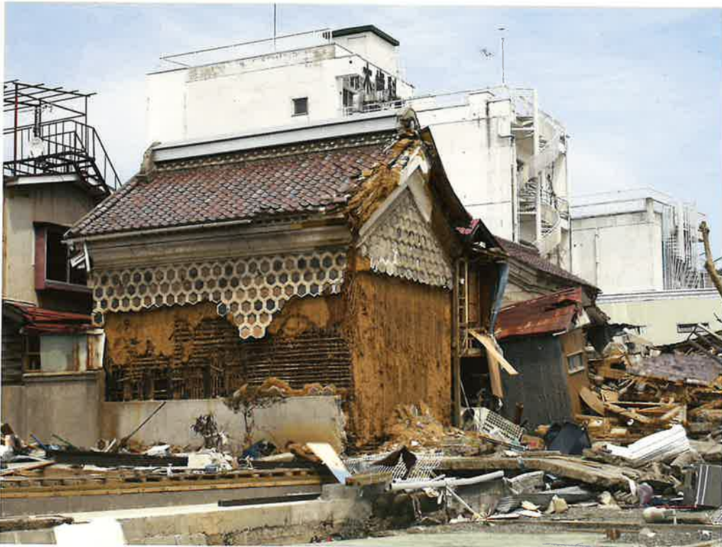
Collapsed buildings (Kesennuma City, Miyagi Prefecture )
