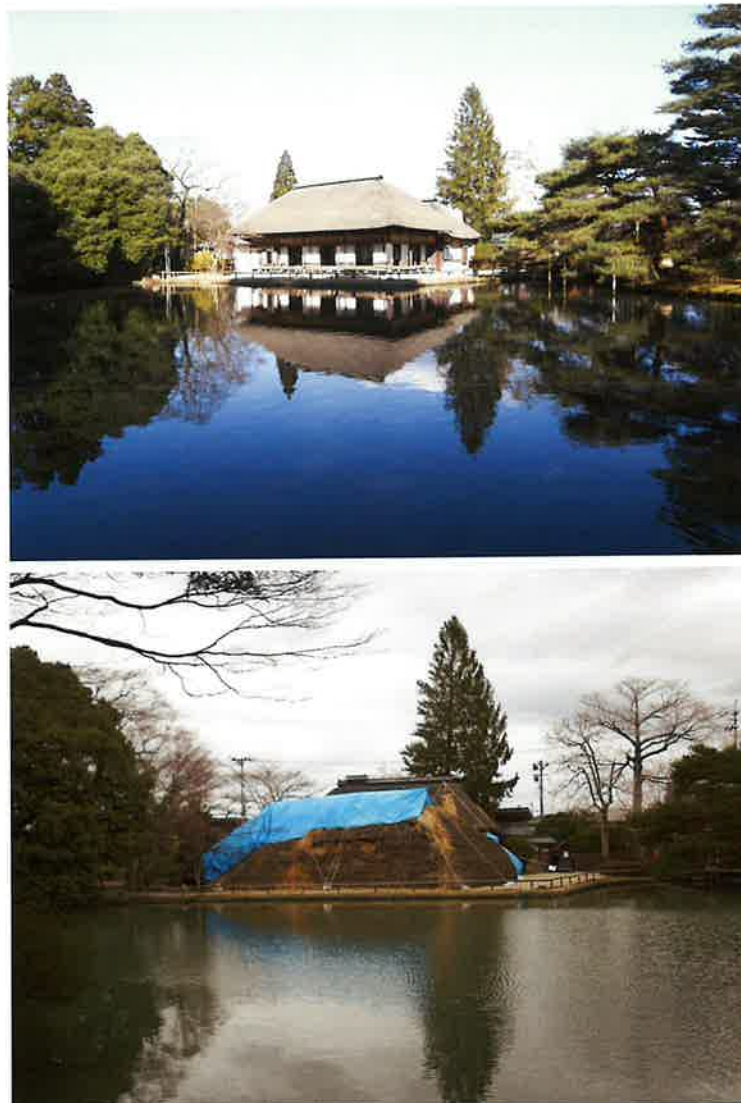
Figure 2.39 Yubikan (Top: Before earthquake; Bottom: After earthquake)
