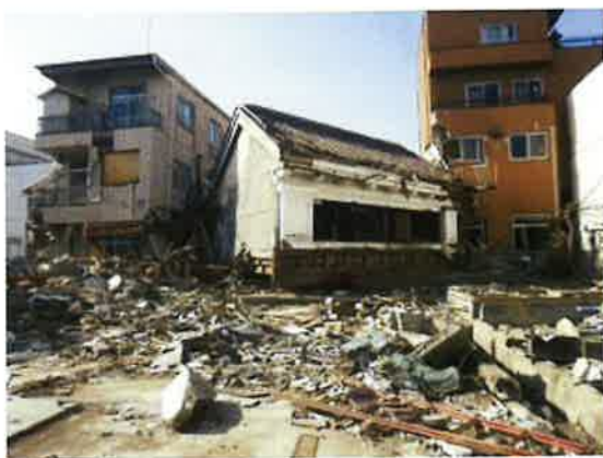
Figure 2.12 The registered tangible cultural property, the Kakuboshi shop, which was swept away by the tsunami
