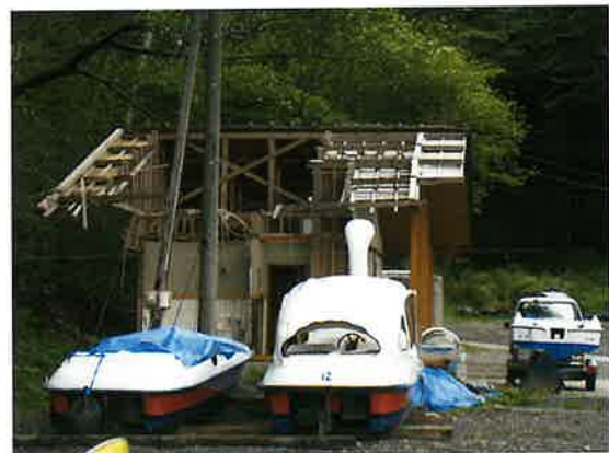
Figure 2.35 Facilities destroyed by the tsunami (Jodogahama)
