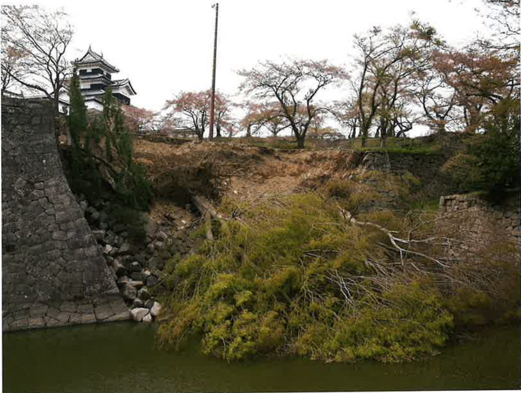
Figure 2.29 Collapsed masonry walls of Komine Castle
