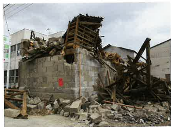
Figure 2.14 Collapse of stone storehouse in Makabe, an Important Preservation District for Groups of Traditional Buildings
