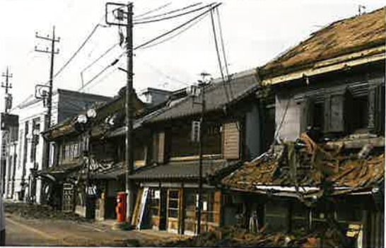
Figure 2.27 Traditional buildings in Sawara (Top: Before earthquake; Bottom: After earthquake)
