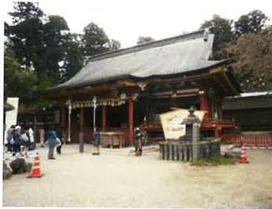
Figure 2.17 The Shiogama Shrine, an important cultural property: Undamaged
