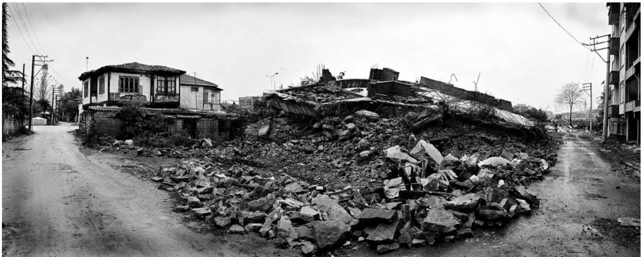
Fig. 4 Surviving humiş house next to a row of collapsed reinforced concrete buildings, Adapazari, Turkey, 1999 (photograph © Randolph Langenbach)
