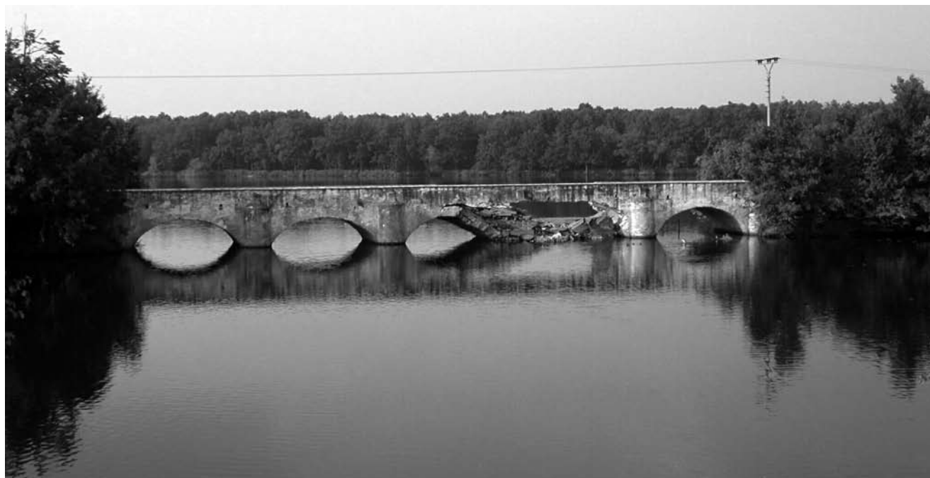
Fig. 4 Stará Hlína, the Inundation Bridge, a masonry bridge from 1781, historically located in the Třeboň pond system. Part of the bridge collapsed; it is necessary to reconstruct the bridge pillar as well as two bridge spans.
