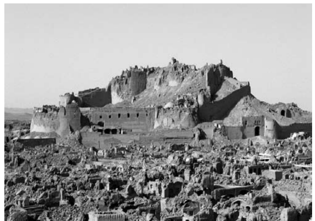
Fig. 2. The Arg-e-Bam, exactly the same view after the earthquake (photograph © Randolph Langenbach)
