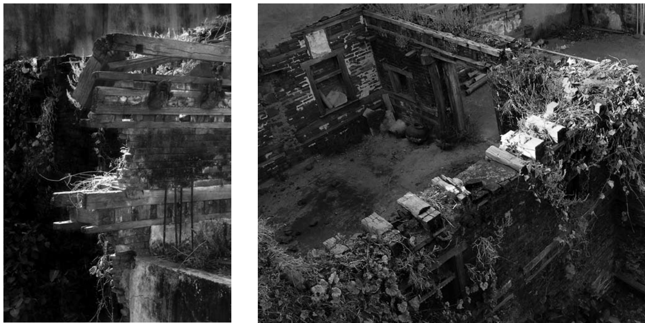
Fig. 9 and 10 Views of ruins of a house in the walled city of Ahmedabad, showing a form of timber lacing similar to that found in taq construction in Kashmir. In the partially dismantled building, the construction with runner beams tied together with cross-timbers pegged to the beams is visible (photographs © Randolph Langenbach)
