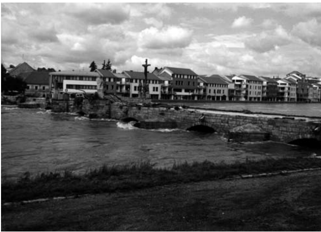
Fig. 5 Písek, the oldest medieval stone bridge in Bohemia from the period after 1250 with Baroque sculptural decorations. The bridge was completely under water, the breastwork walls made of granite square stones and one copy of the Baroque statues collapsed because of the flood.
