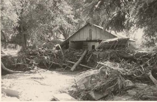
Damages caused by storms
