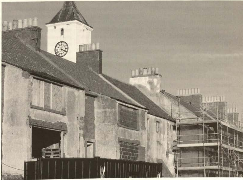
West Wemyss village, Scotland, during restoration
