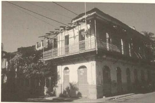
Damages caused by storms
