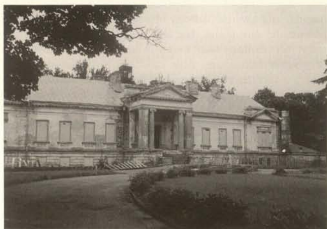
Palace of the estate of Gelgaugiškis, Šakiai district (late 19th century)
