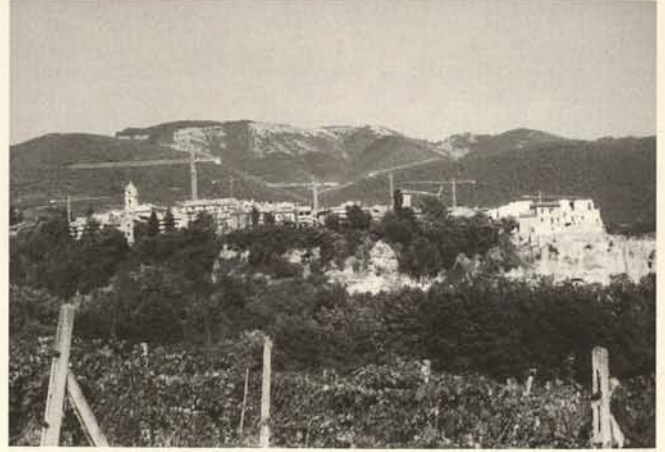
Massa Martama: The town, badly affected by the earthquake, is being repaired
