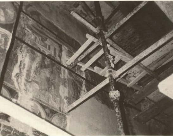
Petkovica Monastery, conservation work on mural painting
