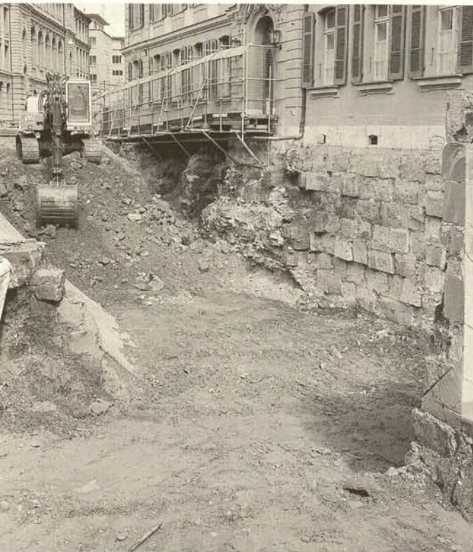
Bern, Waisenhausplatz. The excavation pit for the underground car park goes right up to the walls of the Waisenhaus.
