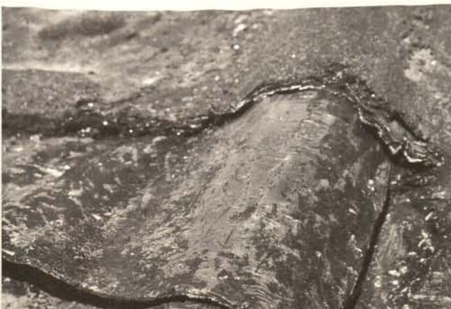
Lead plates covered with bituminous felt
