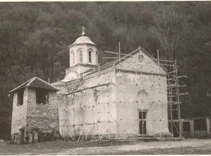
Village of Ba, church of St. Elijah during the conservation works
