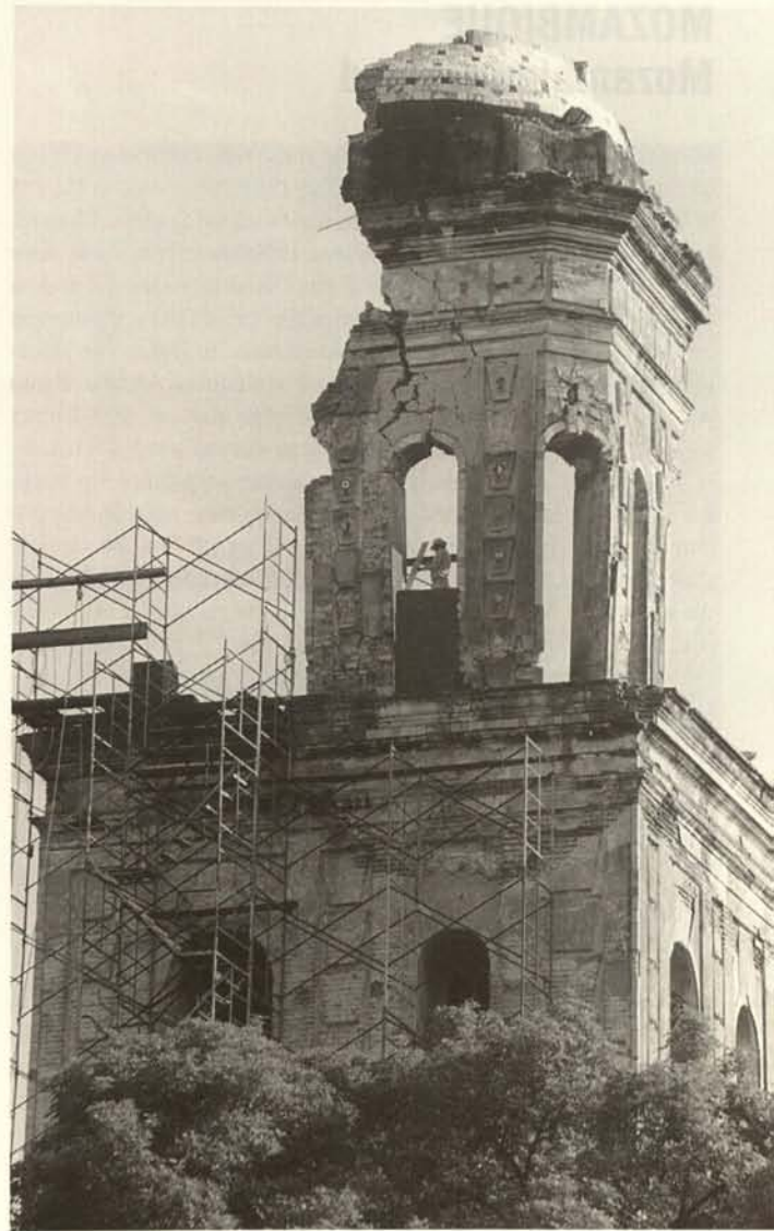
Tower of San Augustin in Puebla after the earthquake of 1999 (see also Heritage at Risk Report 2000 )
