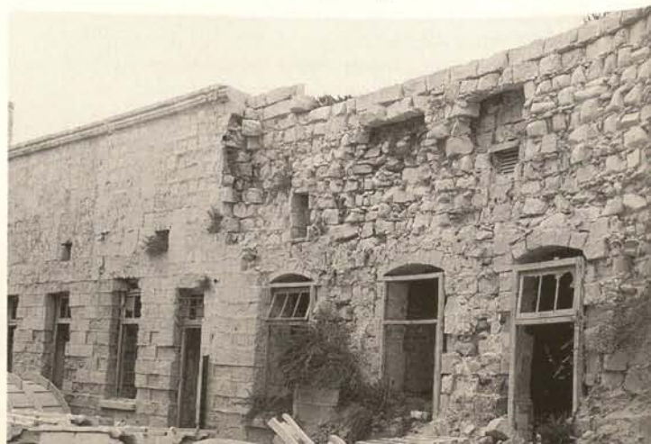
Fort Ricasoli (1670–1900), severely damaged magazines
