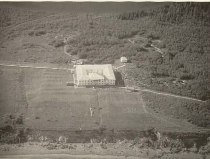
Bird's eye view of York factory depot and shoreline erosion
