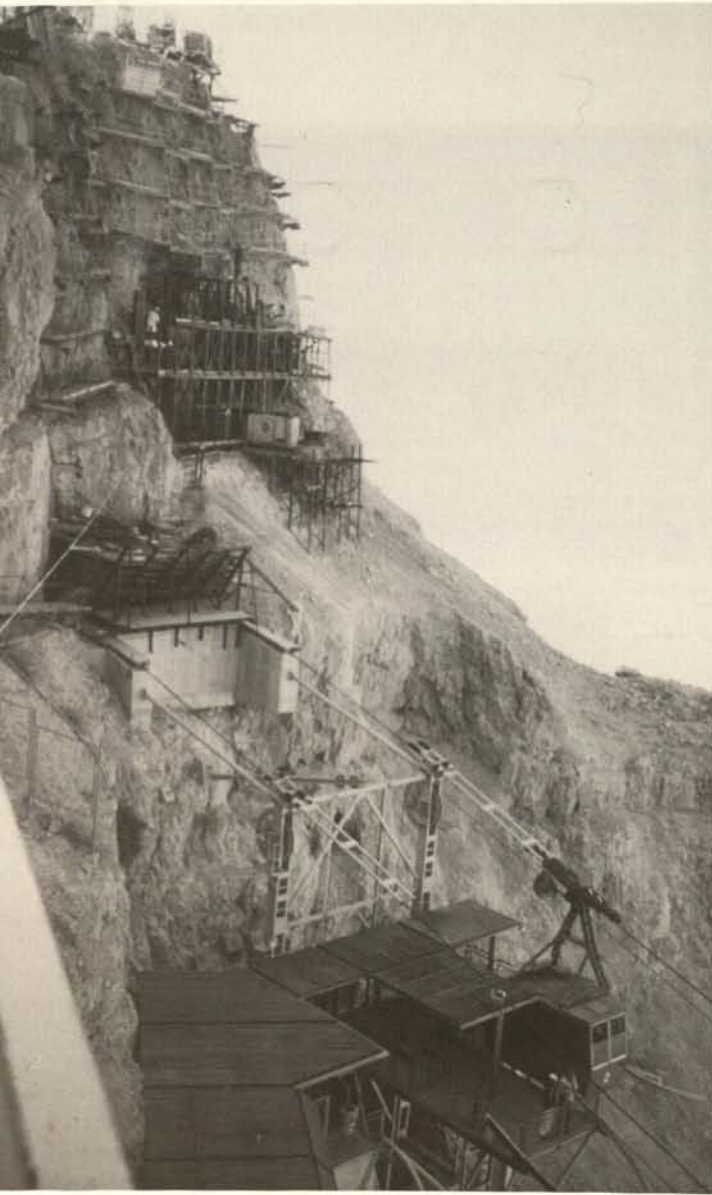
Masada, construction of a new cable car
