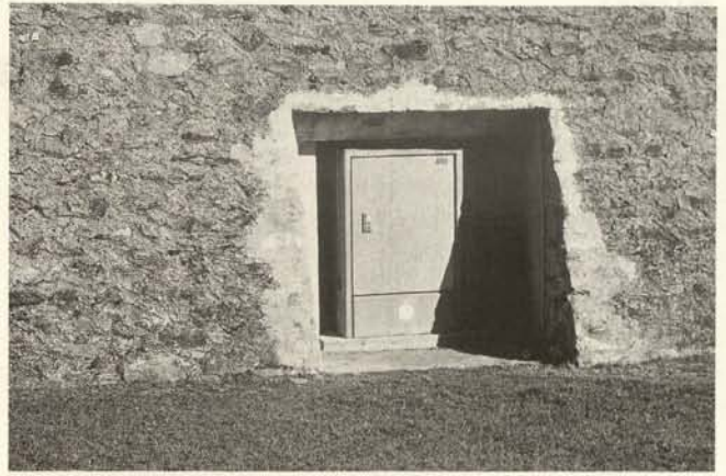
Bellinzona, Castello Grande. Retaining wall with electricity box.
