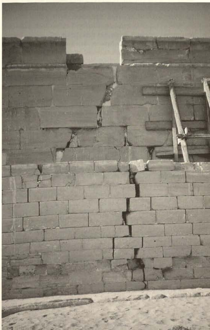
El-Charga Oasis, Hibis Temple, northern wall with ancient crack, mortar from the restoration of 1910-12
