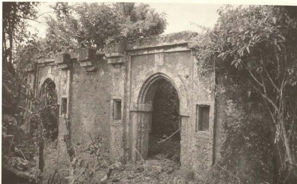
Mwana, remains of a residential house
