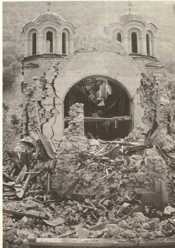
Cathedral Church of St Atanasie, Lesok village, after damage
