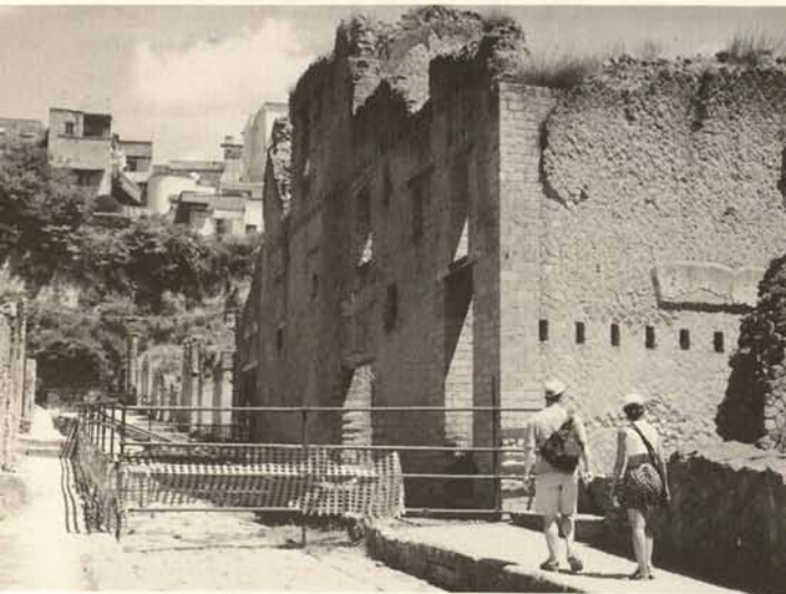
Herculaneum, 5th Cardo with street front of the vestibule of the Palestra in danger of collapse
