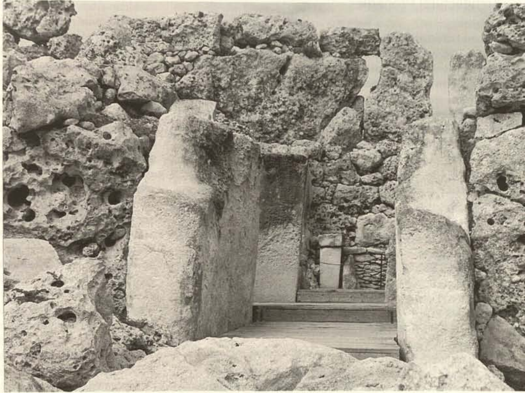
Ggantija Temples (Neolithic), structural instability and collapsing in parts
