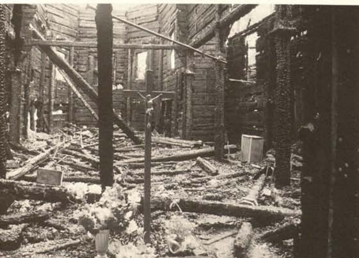
Among the principal dangers mentioned in last year's report (see Heritage at Risk Report 2000 , p. 155) is fire hazard threatening wooden buildings. A sad example is the recently burnt down wooden church of St Anne (17th century) in Długa Koscielna (Halinow); here the state before and after the fire.
