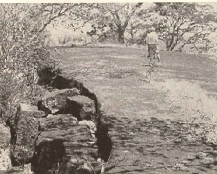
Blocks of tuffaceous layer breaking off as a result of erosion in the underlying soil layer at El Muerto
