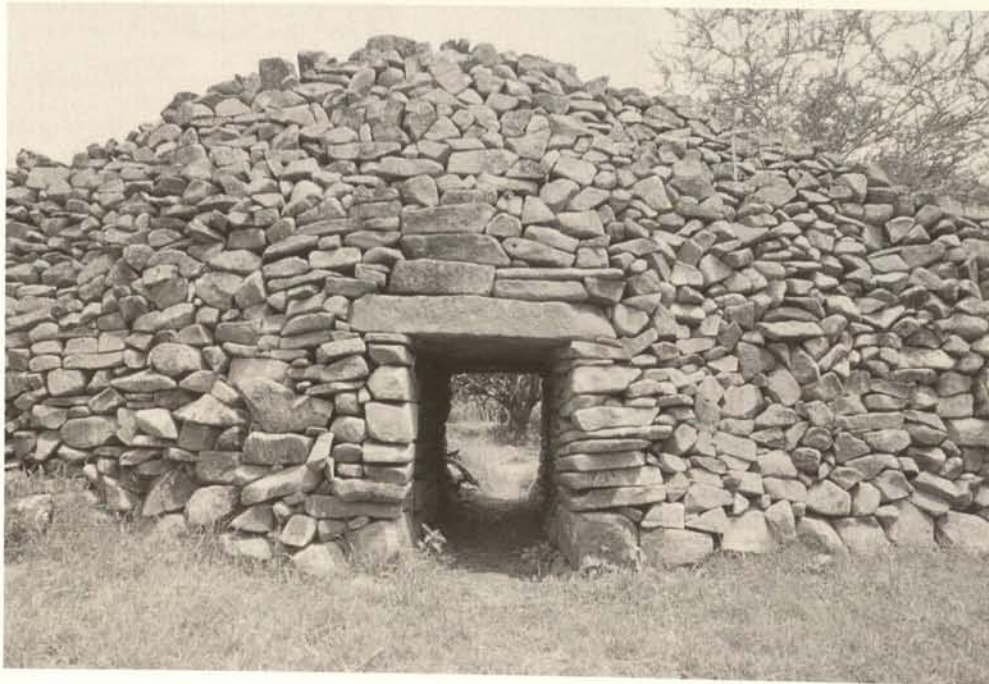
Entrance of dry-walling enclosures of Thimlich Ohinga in South Nyanza. Note the similarities with Great Zimbabwe.
