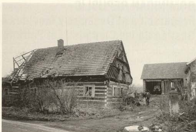
Studeňany, land-register No. 45, District of Jičín - a dilapidated timbered farm before its complete demolition
