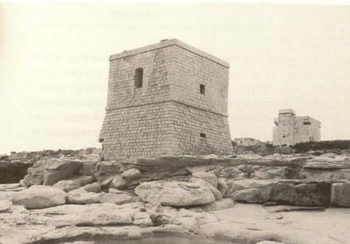
Coastal tower (c. 1658/59), damaged by natural processes
