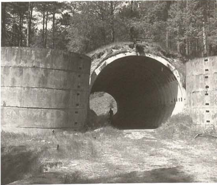
Brzeznicza, near Borne Sulinowo, example of a Soviet military structure for missiles from the Cold War
