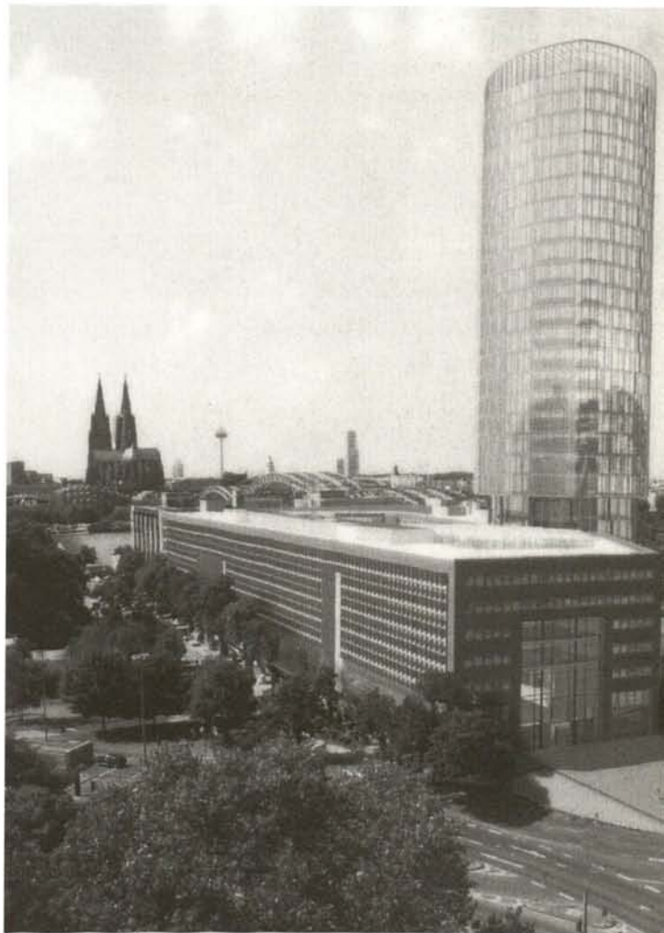
Cologne, project for the RZVK high-rise building with view towards the cathedral (computer simulation: Data Services GmbH)
