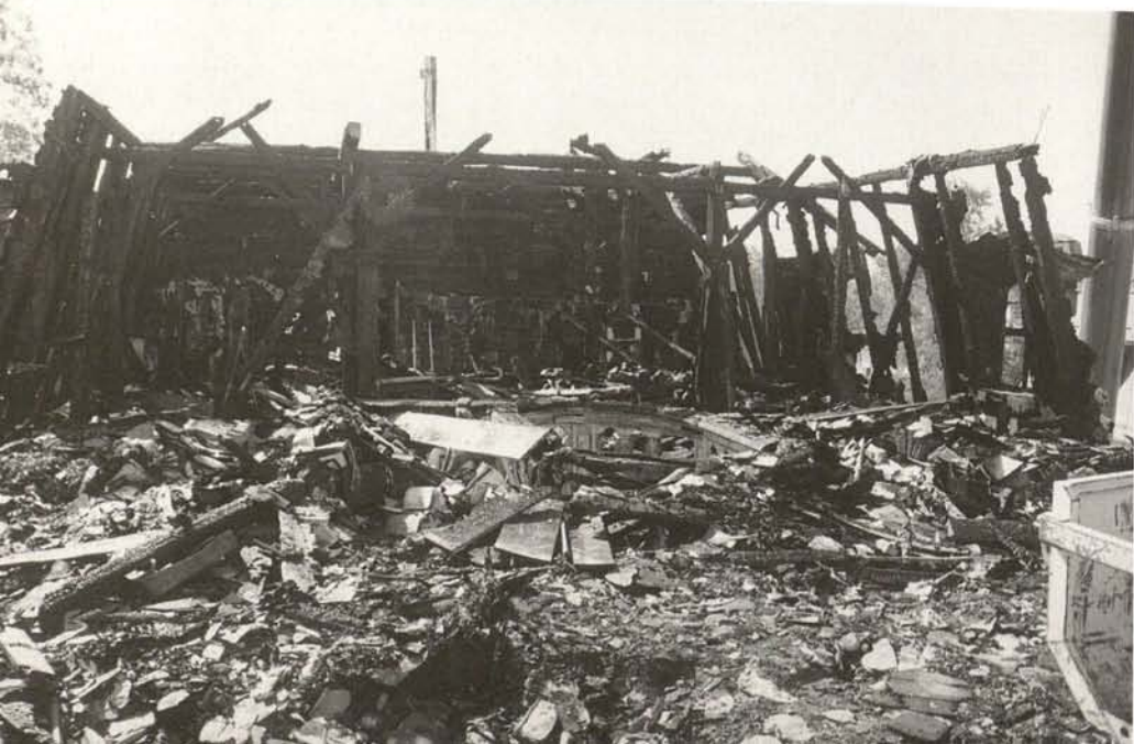
Top storey of the library building on the day after the fire. On the floor burnt shelves and books (photo: J. Seifert)
