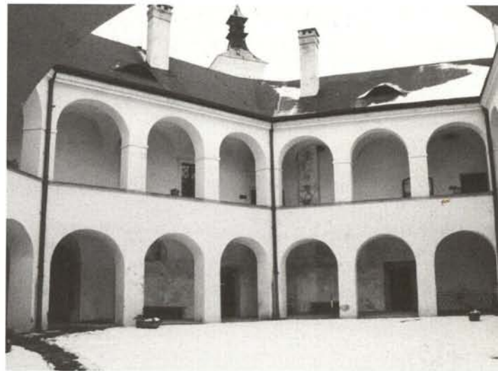
Roztoky, the manor house, the main building courtyard
