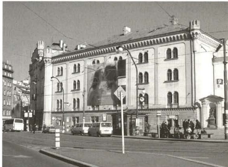
Prague, the historic Josefská Barracks from Republiky Square. The vacated building is ready for demolition. Only the façade is to be preserved.
