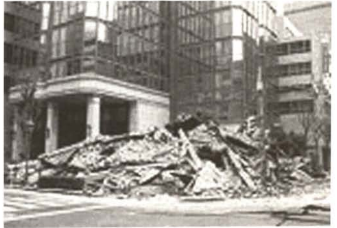
Kyokoryuti 15 banken, destroyed by earthquake
