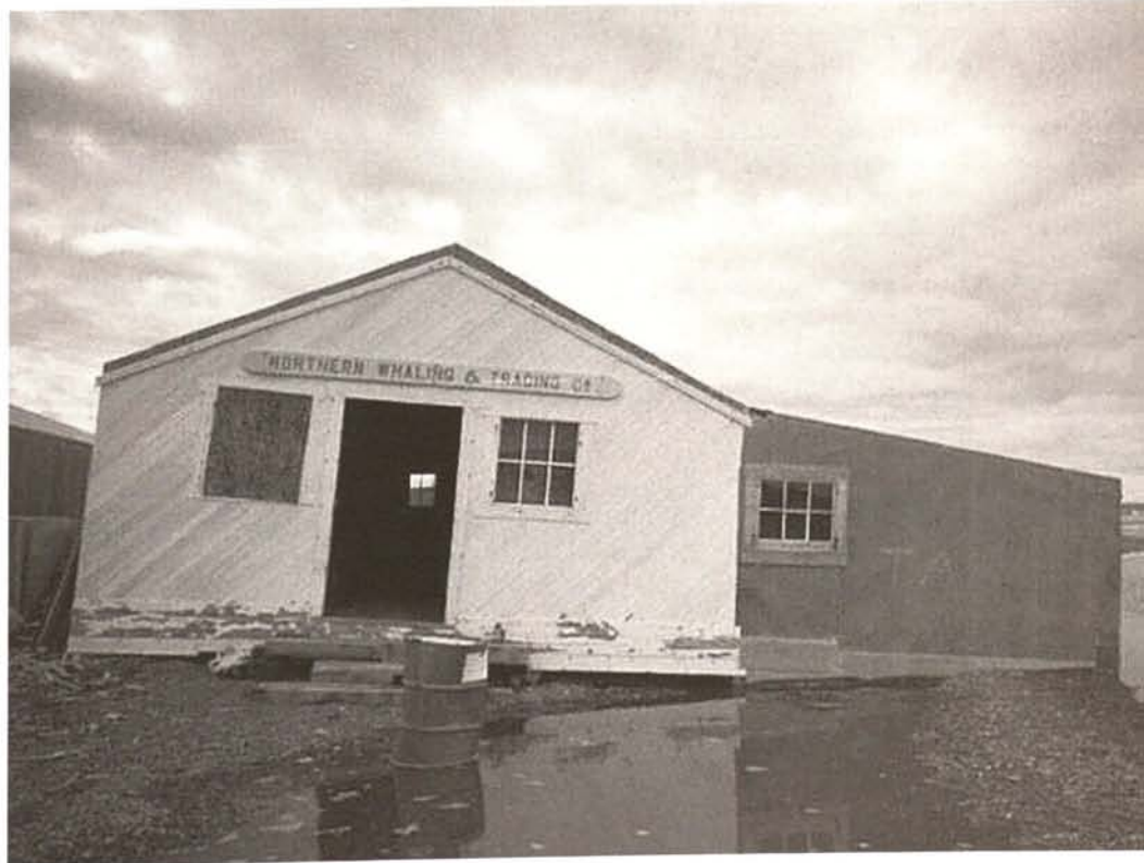
Northern Whaling and Trading Company Store, Pauline Cove, Western Canada Arctic, prior to dismantling of shed addition in 2000
