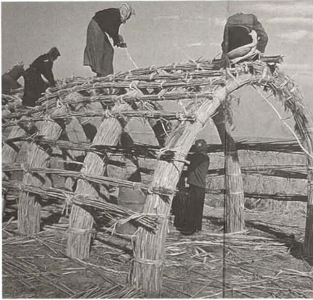
Reeds house under construction
