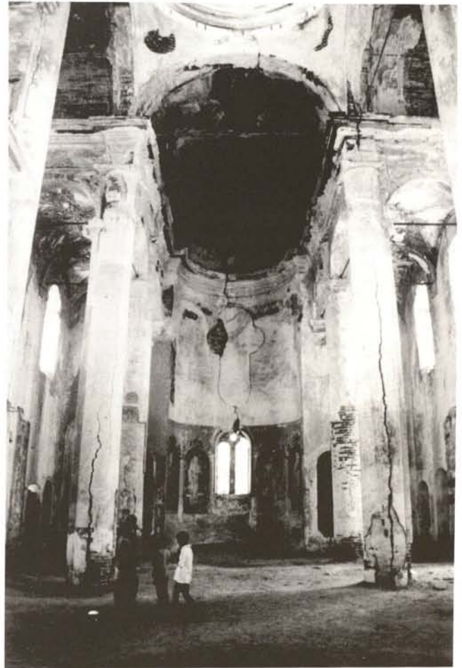
Cunda Adası, near Ayvalık, domed church, cracked brick-pillars and vaults
