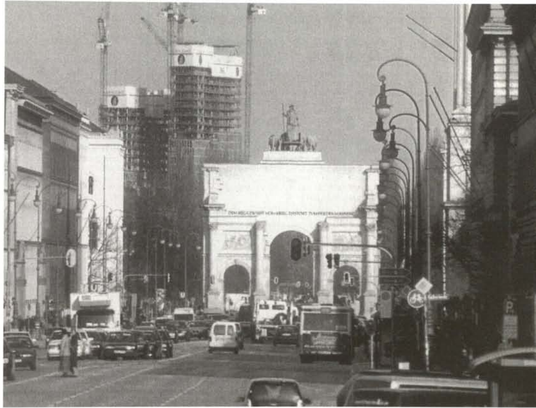
Munich, Ludwigstrasse with triumphal arch and the so-called Munich Highlight Towers under construction, February 2004 (photo: Heinz Gebhardt)
