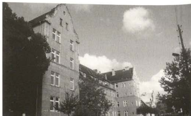
Quedlinburg, former infantry barracks, erected in 1909, buildings in Gneisenaustrasse, October 2004 (photo: A. Hubel)
