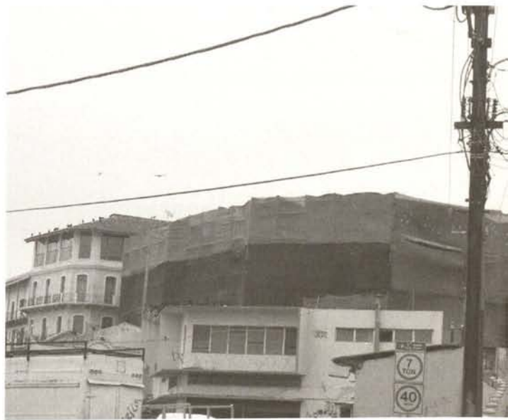
The demolished facades covered in plastic
