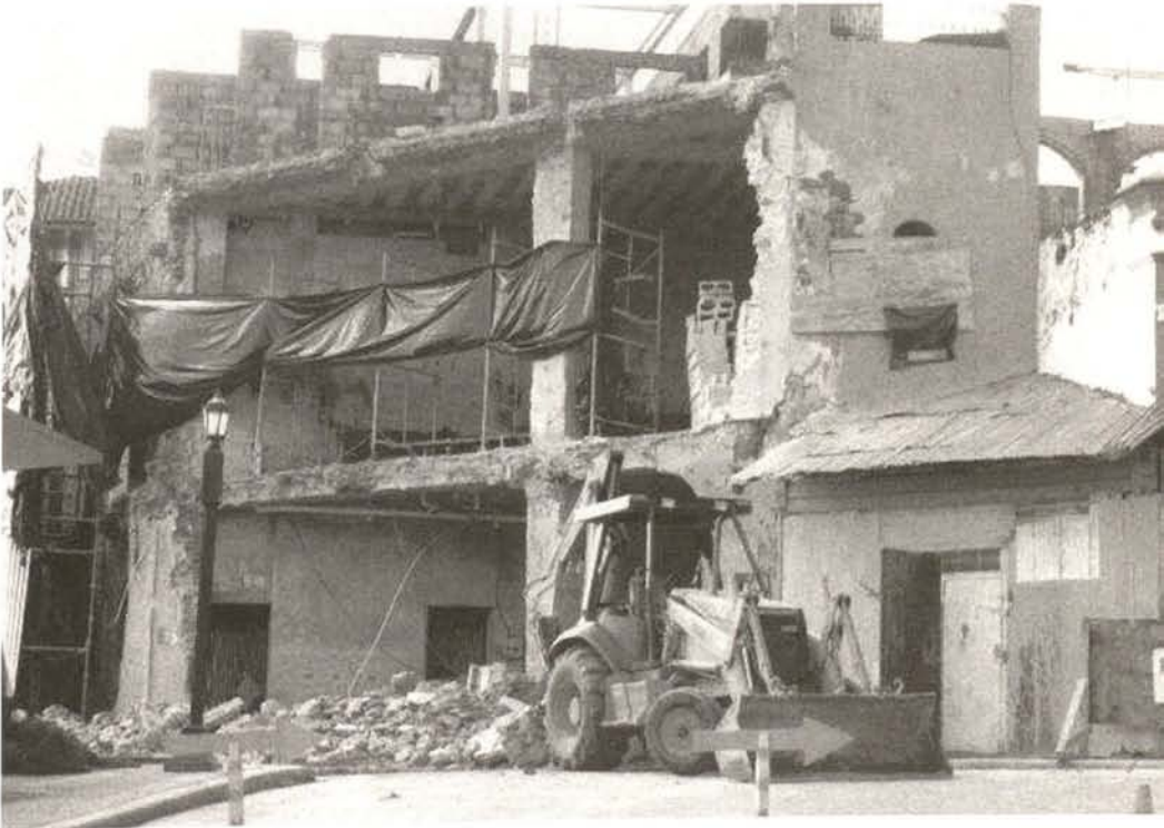
The demolished facades covered in plastic
