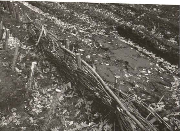
Kratochvíle, foundation of willow wattles on the bank of the brook near Kratochvíle
