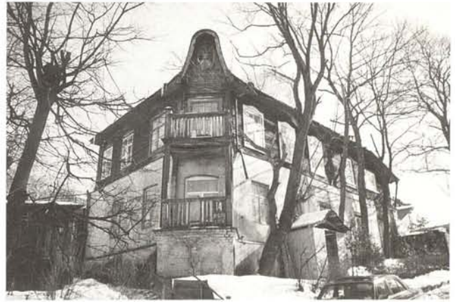
House in Pavasario Street
