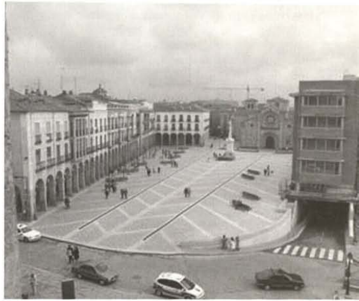
Avila, Plaza de Santa Teresa (Mercado Grande), on the right new building 'A' with entrance to the parking area
