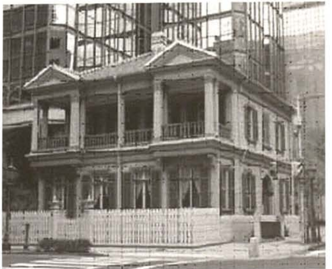
Kyokoryuti 15 banken, in process of reconstruction
