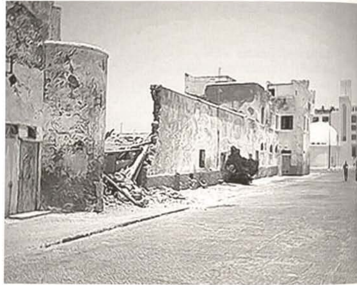
Demolition of a wall of the fort
