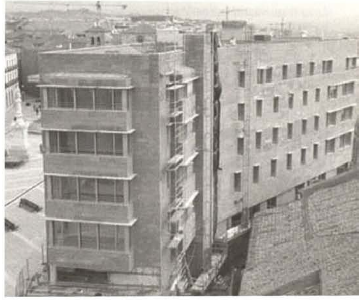
Avila, building 'A' by Rafael Moneo, rear side
