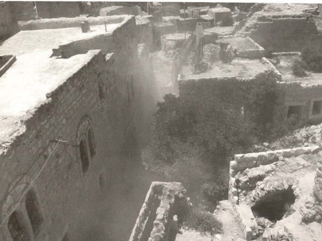
Destruction of Mamluk-era houses for settlers' road through Hebron's Old City
