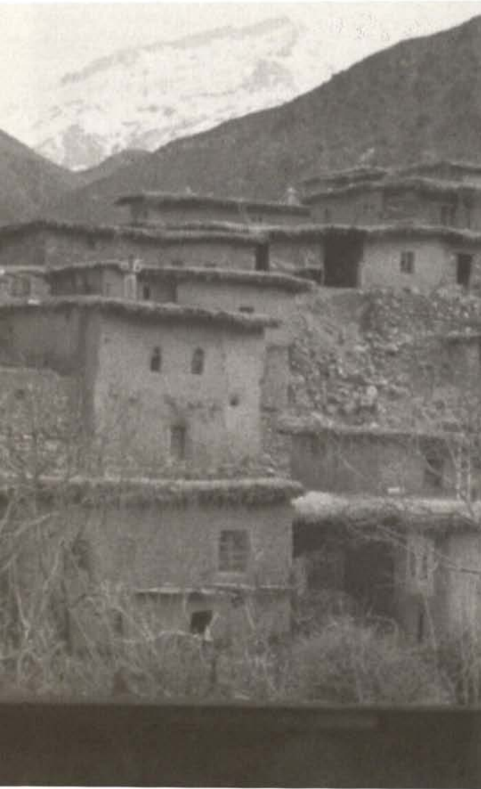
House in Haj Omran, North Iraq, built of stone and mud bricks (photo: Nik Wheeler)
