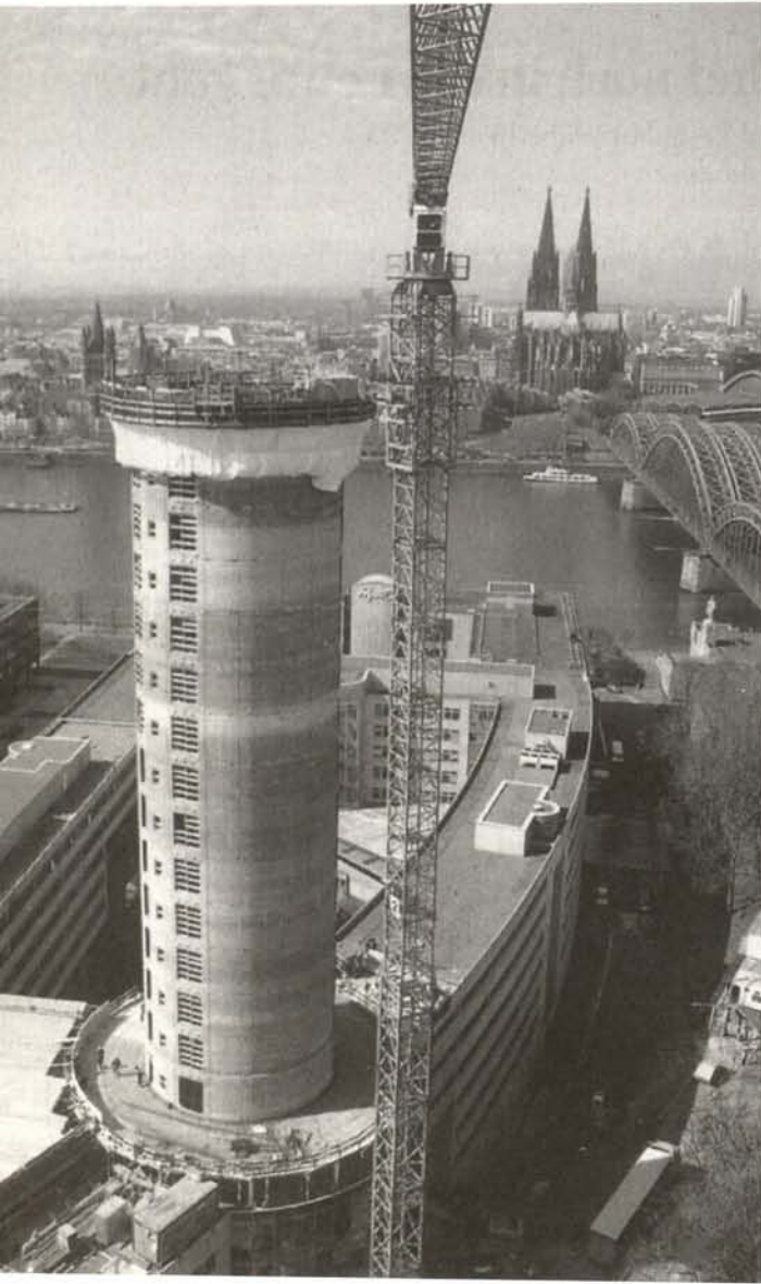
Cologne, the RZVK building during construction
