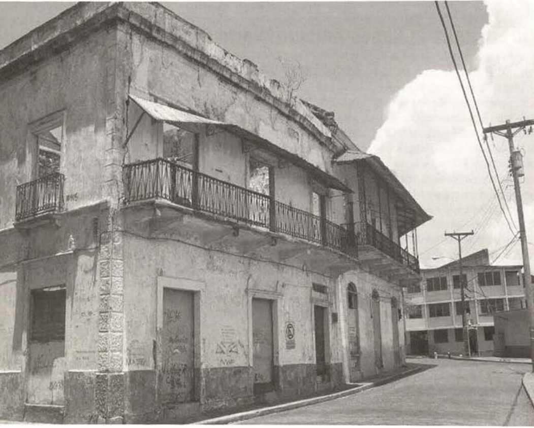
Ave. Eloy Alfaro, facade (demolished)
