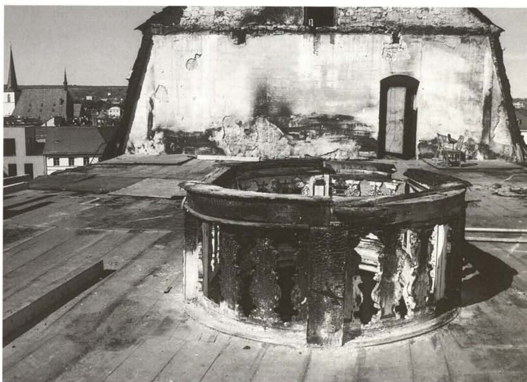
The cleared-out top storey of the library (photo: J. Seifert)
