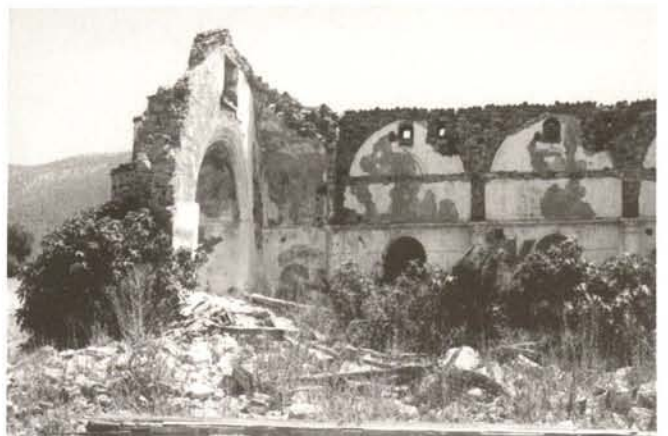
Yayla Köyü, area of Muğla (Caria), village church (19th c.): View from the north
