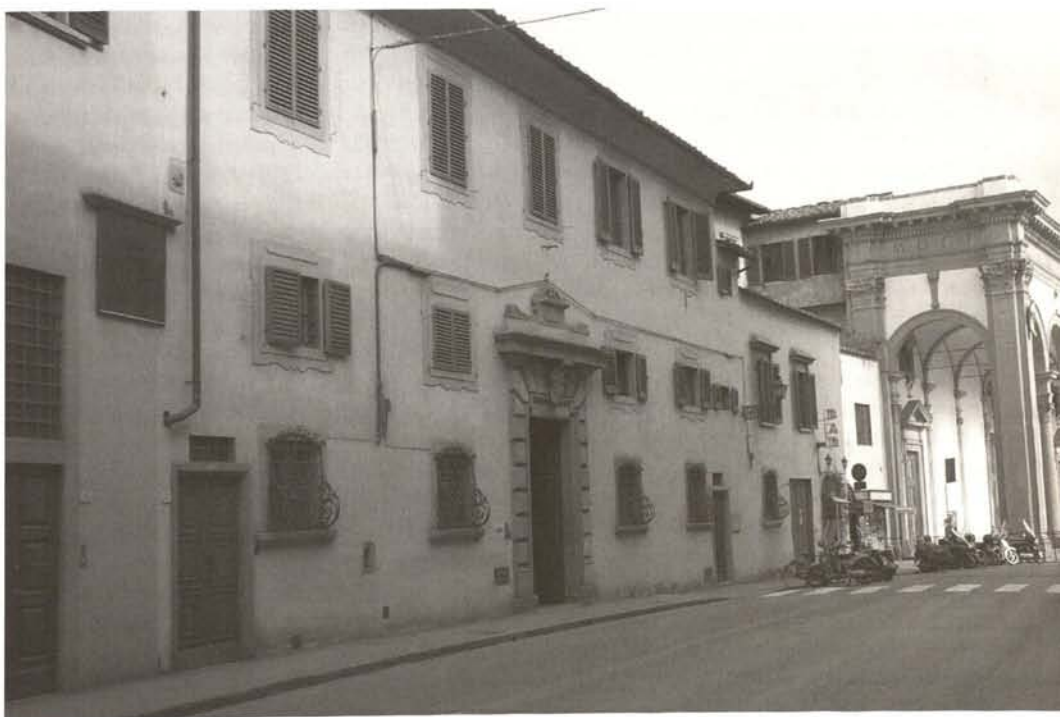
Florence, Via C. Battisti near Piazza della SS. Annunziata (example of building at risk of sale)
