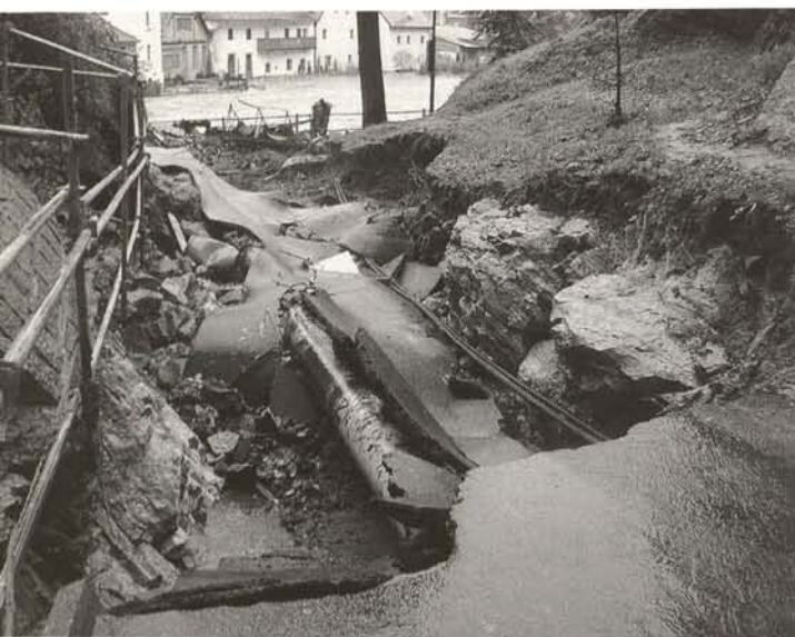
Ceský Krumlov, the condition of the access road under the Plášťový Bridge after the water falling off
