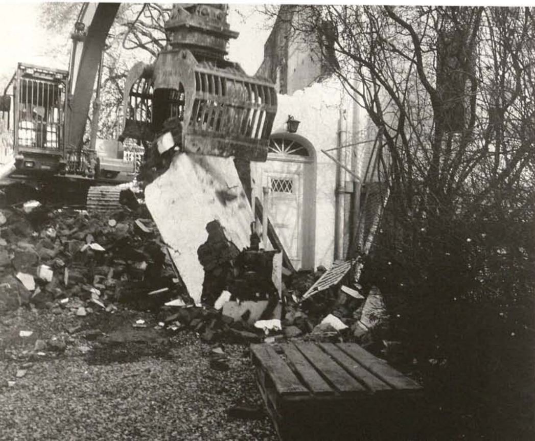
Demolition of the museum, on the left the former entrance
