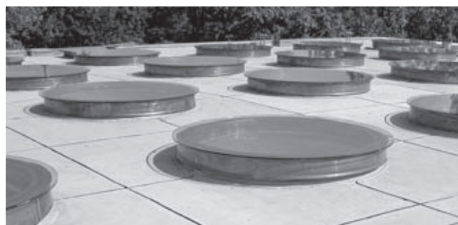
Viipuri Library, 1927–35, arch. A. Aalto. Rooflights before and after the restoration in 2003
