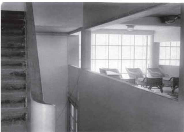
Narkomfin commune house of the Ministry of Finance on Novinsky Boulevard 25, Moscow, arch. M. Ginzburg, I. Milinis, 1928–30. Interior of the communal block. 1930
