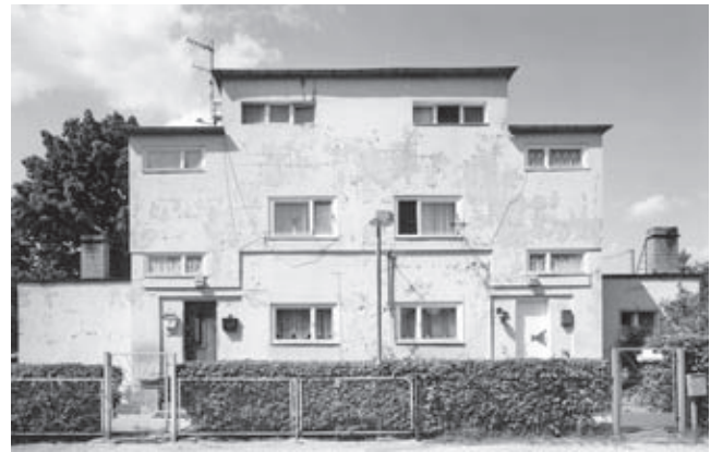
Settlement „Neu Jerusalem“, Berlin, 1923–24, arch. E. Gutkind. Current Condition
