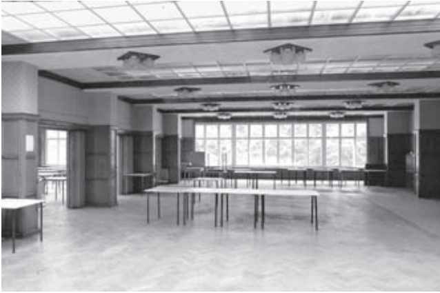
Former school of the German Trade Union (ADGB) in Bernau near Berlin, refectory before the reconstruction, 1998
