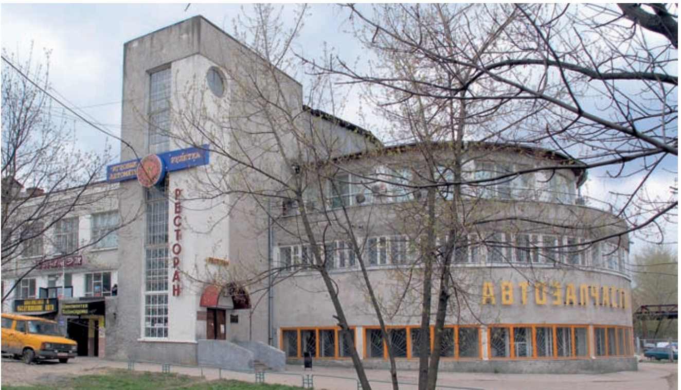
Metal workers club in Kashira near Moscow. 1929–30, arch. unknown. Current condition. Credit: I. Chepkunova, Moscow
