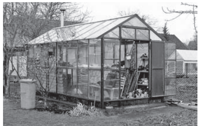
Alteration of an original steel window: greenhouse, restoration of the window, window after re-installation
