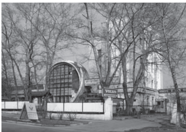
"Gosplan" – garage of the State commission for planning, Aviamotornaya street 63, Moscow, arch. K. S. Melnikov, 1933–36, monument of local importance. Condition in 2005
