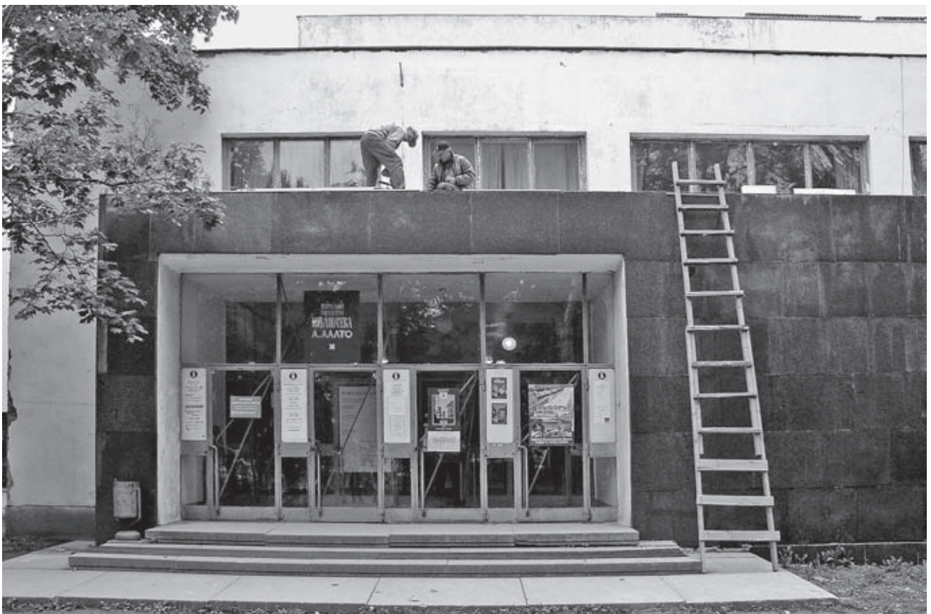
Viipuri Library, arch. A. Aalto, 1927–35. Main entrance during restoration works in 2003
