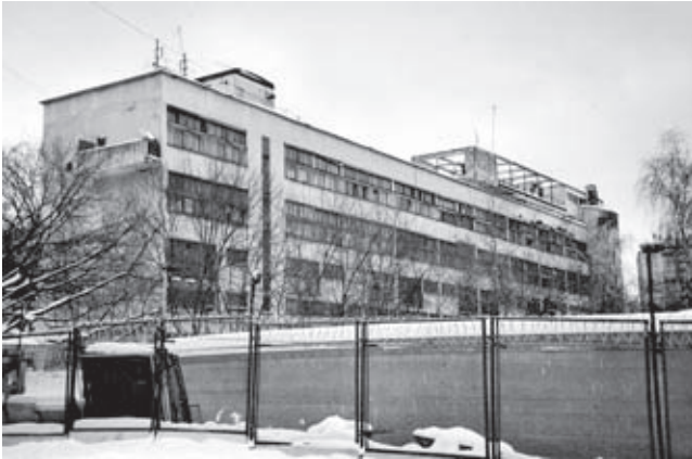
Narkomfin Building in Moscow, arch. M. Ginzburg, I. Milinis, 1928–30. View from the west in 2003
