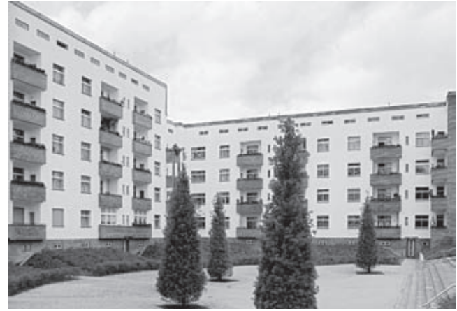
Housing block Ernst-Fürstenberg-Strasse, courtyard, after restoration, 1998
