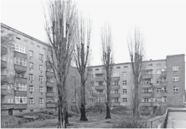
Housing block Ernst-Fürstenberg-Strasse, courtyard, before restoration, 1997
