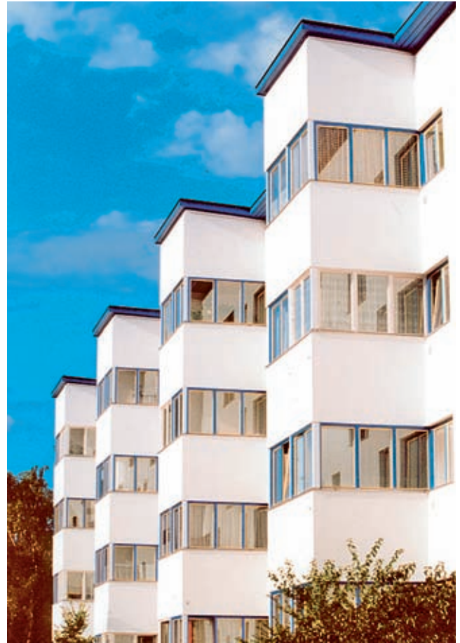
Weiße Stadt (White City), Berlin-Reinickendorf, 1929–31, arch. B. Ahrends, L. Lesser et al. Current condition. Credit: Winfried Brenne Architekten, Berlin
