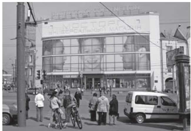
Mostorg department store, Krasnaya Presnya 48/2, Moscow, arch. A. A. Vesnin, I. A. Vesnin, V. A. Vesnin, 1929, monument of local importance. View from the square in 2005. The transparent façade is now an advertisement board
