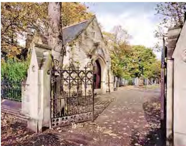
Fig. 4 Southern Cemetery, Manchester, entrance gates and Gothic Revival Ohel in the Jewish section (Photo: Tony Perry © English Heritage)
