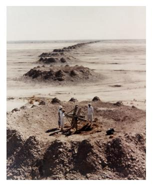
Fig. 2 Qanat system in Iran (Source: International Center of UNESCO on Qanat and Historic Hydraulic Structures).
