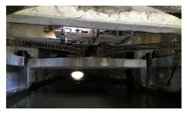
Fig. 5 1980 reconstruction of the closing doors in the underground canal under Nieuwmarkt, Amsterdam. The canal functions as a connection, eventually transporting water discharge from the Amstelland catchment in the direction of the North Sea. The closing doors protect the city from flooding when outside water levels are high (Source: Maarten Ouboter).
