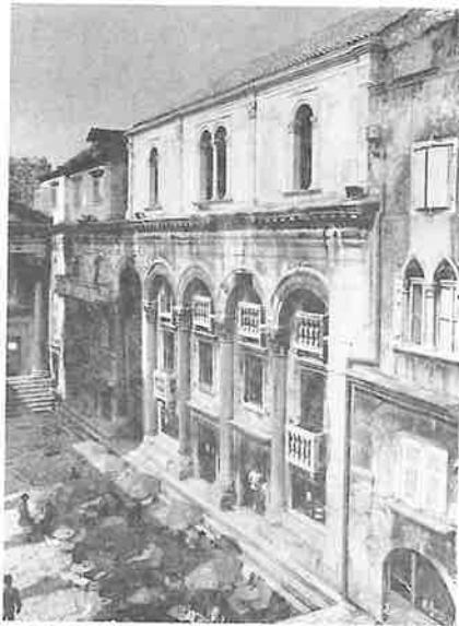
Fig. 7. Western side of roman Peristyle, an example of reuse throughout centuries.
