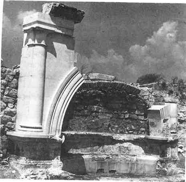
Fig. 4 a and b. Complementary Form - Restoring the continuity of original fragments. Nymphaeum. 2nd century. Preserv. 1970. Tac Gorsium Hungary.
