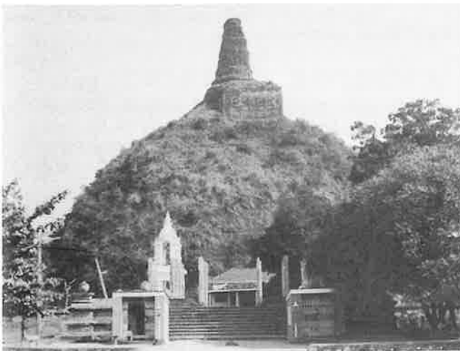
Fig. 4b. A portion of stupa cube has callapsed.
