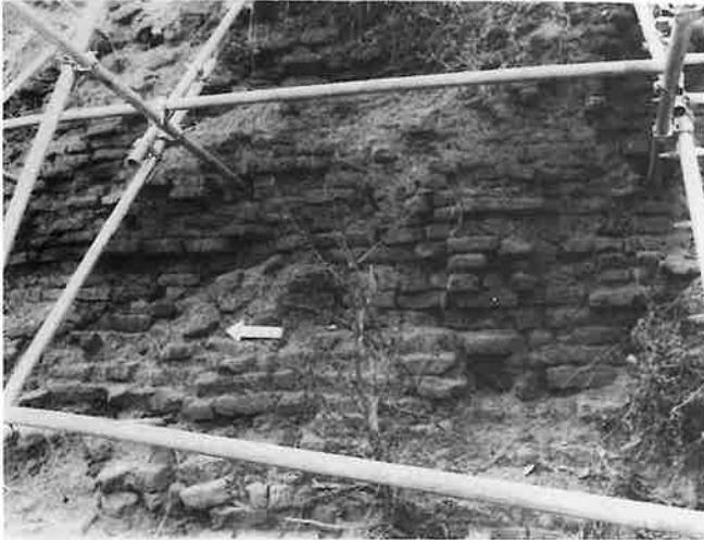
Fig.3 Stupa dome brick surface
