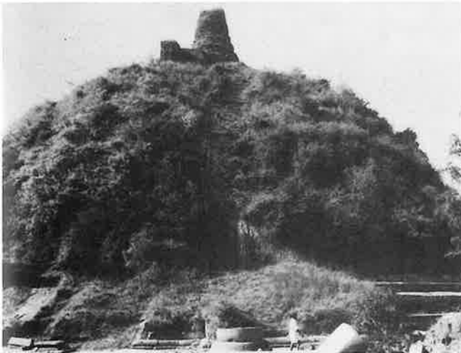
Fig. 4a. A portion at stupa cube has callapsed.
