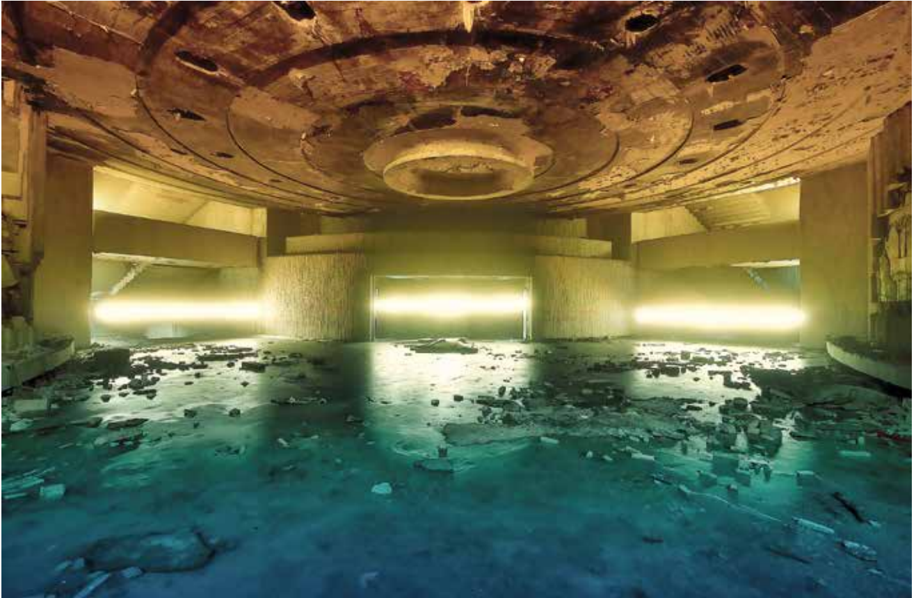
Fig. 5 The foyer at the main entrance
