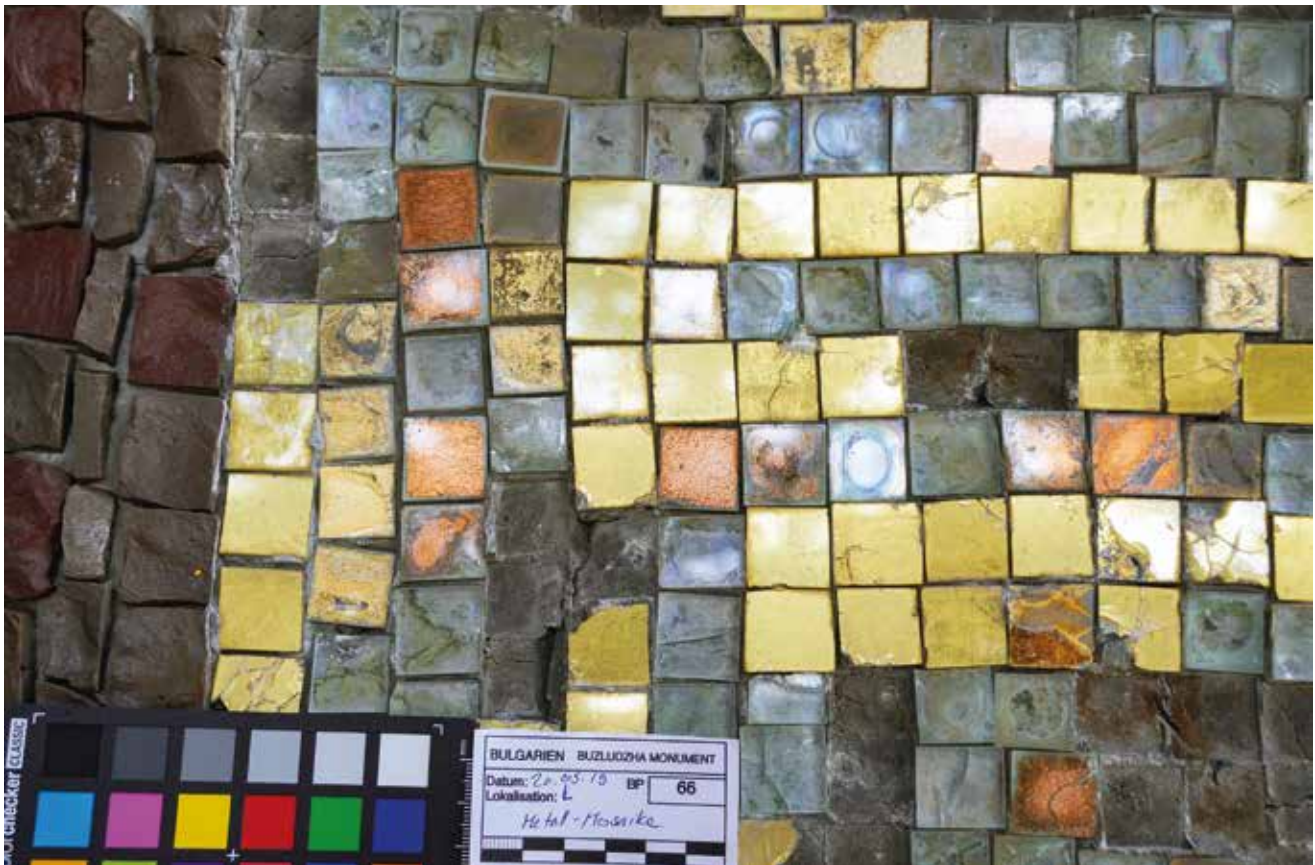
Fig. 7 Main Hall, inner ring, “gold-like” glass mosaic with metal foils of different alloys
