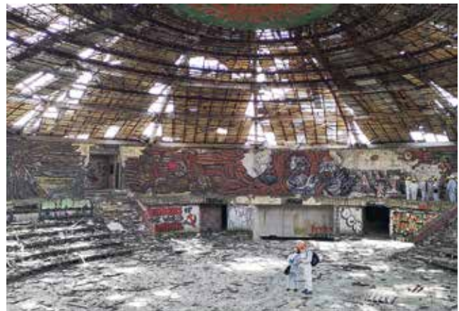
Fig. 9 The interior of the main hall where the inner mosaic ring and the steel roof structure can be seen
