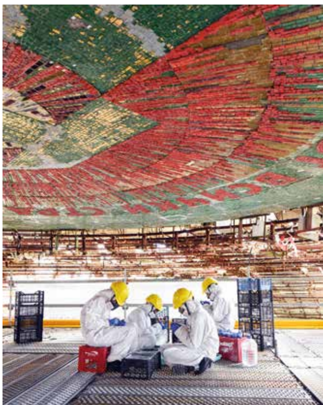
Fig. 16 Stabilisation of the mosaics of the dome
