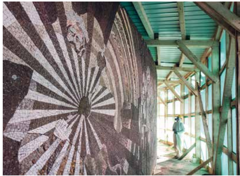
Fig. 10 Shelter erected around the outer mosaic ring
