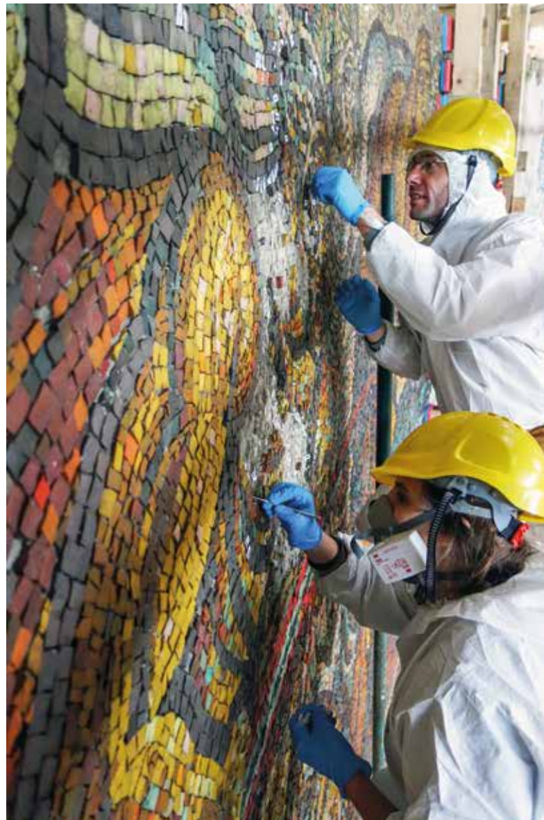
Fig. 7 Emergency measures carried out on the mosaics
