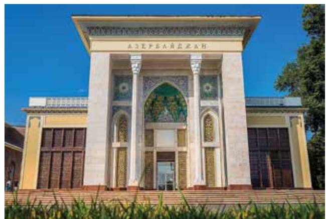
Fig. 6 Pavilion No. 14 (former pavilion of the Azerbaijani SSR) after restoration
