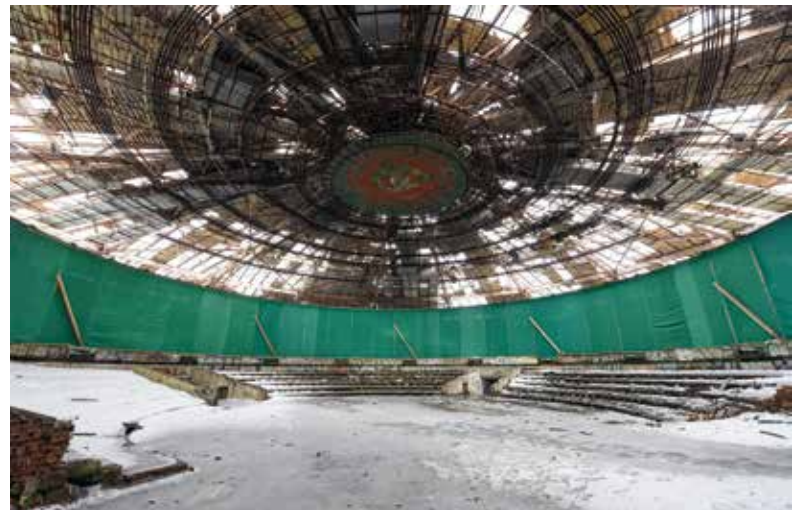
Fig. 3 Main Hall, inner ring after the realized enclosure, 2020
