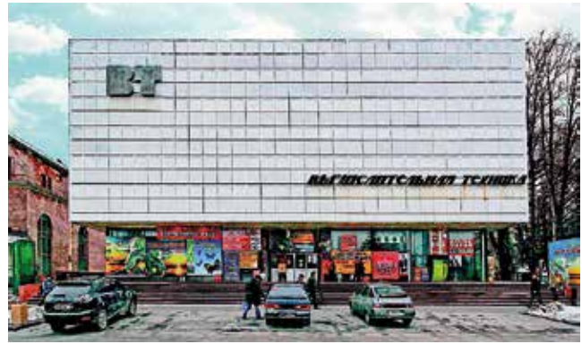
Fig. 4 Pavilion No. 14 (former pavilion of the Azerbaijani SSR) before restoration
