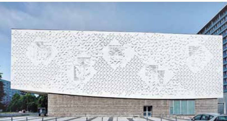
Fig. 5 Berlin Mitte, Kino International, detail of south facade, photo Wolfgang Bittner, 2007
