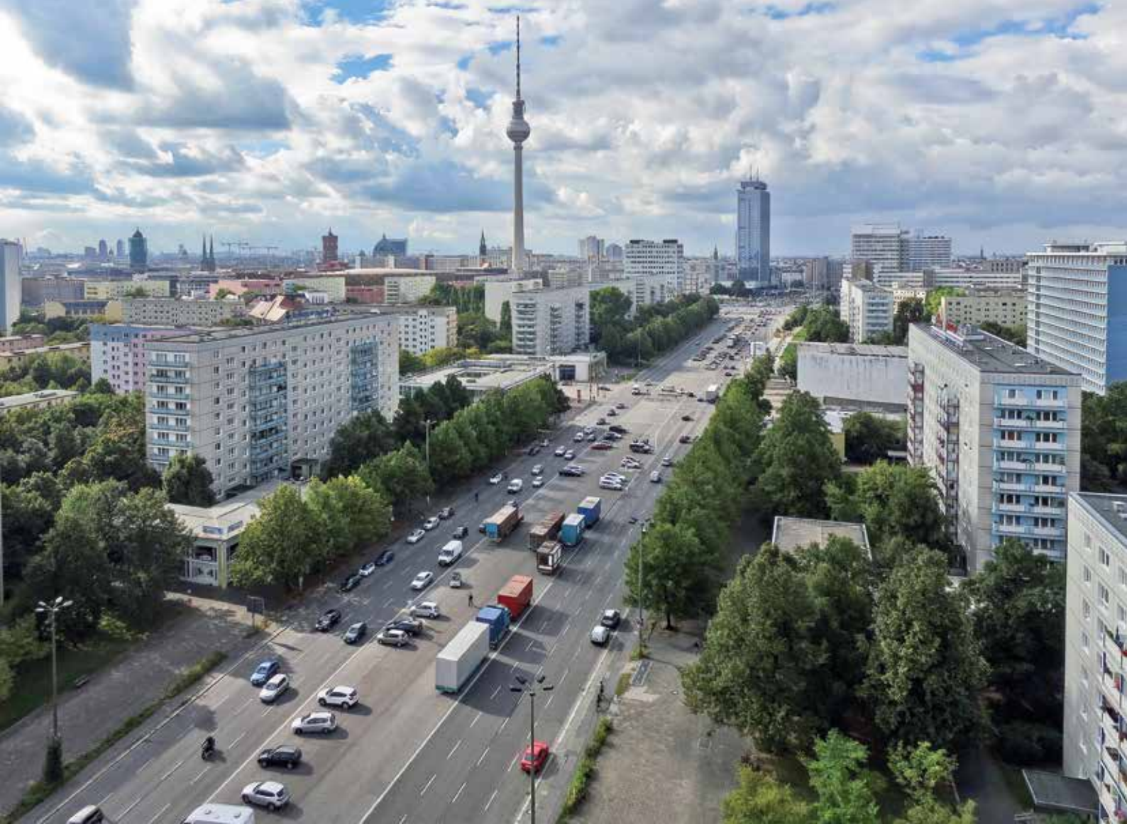
Fig. 2 Berlin Mitte, Karl-Marx-Allee, 2nd construction phase, photo Wolfgang Bittner, 2013
