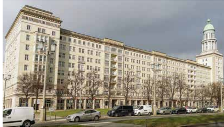
Fig. 4 Berlin, buildings in Karl-Marx-Allee (formerly Stalinallee), photo Hitzfeld, 2018
