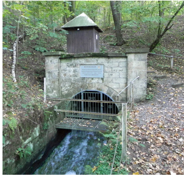
Fig. 3 Water gallery in the Ore Mountains in Saxony, Germany
