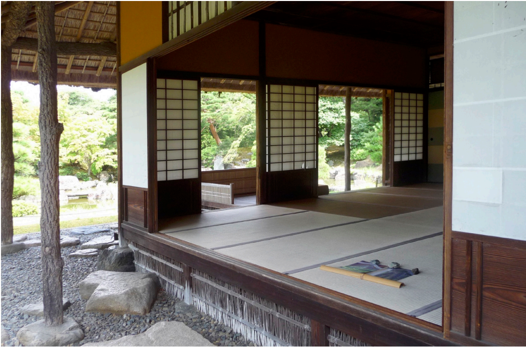
Fig. 3 Detail of tatami flooring in a pavilion, the Shokin-tei, at Katsura Rikyu Imperial Villa in Kyoto, Japan.
