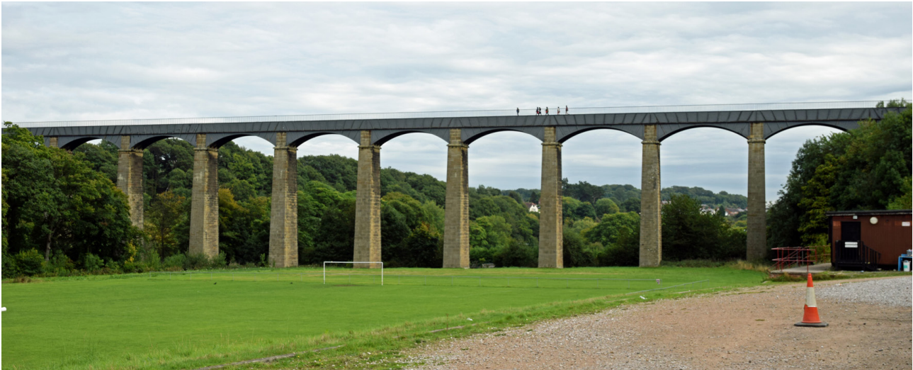
Fig. 5 Pontcysyllte Aqueduct of the Llangollen Canal in Wales, United Kingdom
