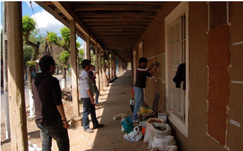
Fig. 27. Workshop in applying mud stucco, Quinta de Tilcoco, San Pedro de Alcántara, O'Higgins region, Chile (Source: SEREMI, MINVU)
