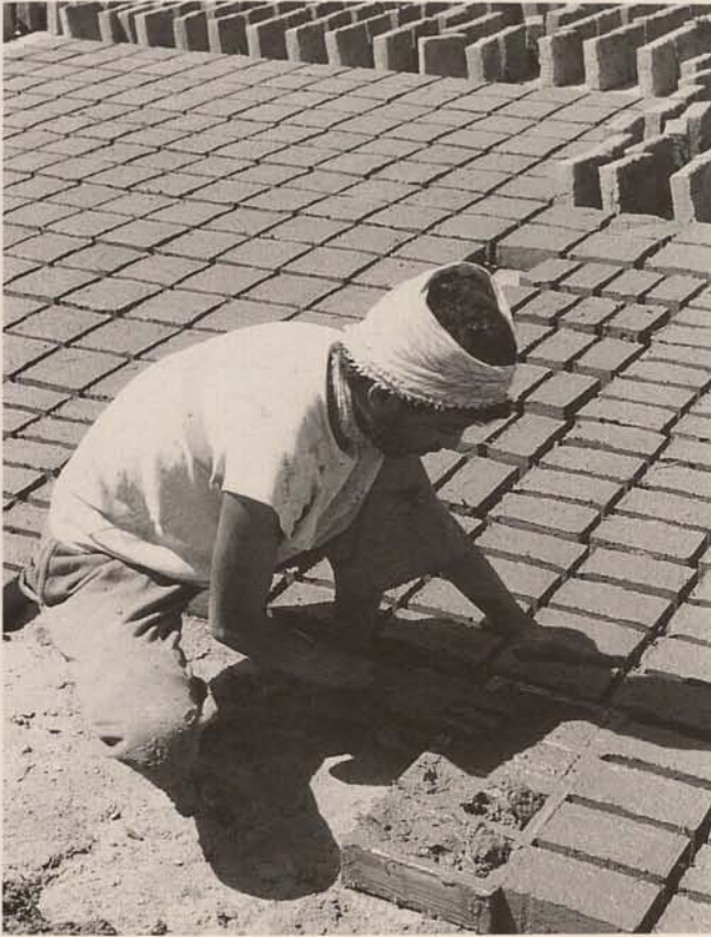
Abb. / Fig. 81. Lehmziegelherstellung in traditioneller Technik, Abstrich und Trocknung / Production of clay bricks according to traditional practice, leveling and off drying
