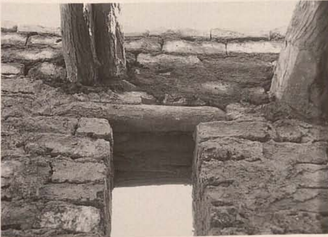
Fig. 92. Reconstructed part of a brick wall with a window, reusing old bricks and round timbers
