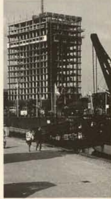
Ill. 1 Rotterdam, Blaak 333 during its renewal (1987-1992)
