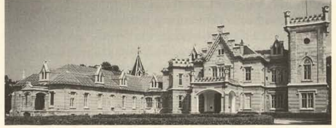
Hungary, Nadasdy Manor House, restored as a conference centre by the Institute of State Care of Monuments in cooperation with the Nadasdy Foundation (description at page 54)
