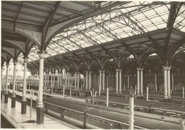
Ill. 1. The interior of the trainshed at Liverpool Street Station, London, designed by E. Wilson, 1874-5, following its refurbishment by Nick Derbyshire.
