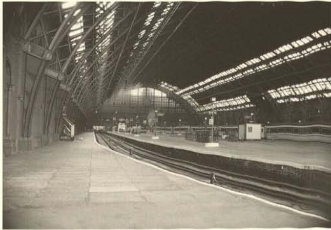
Ill. 2. The trainshed at St Pancras Station, London, by W.H. Barlow, 1868 shortly to become the terminus for Eurostar trains.
