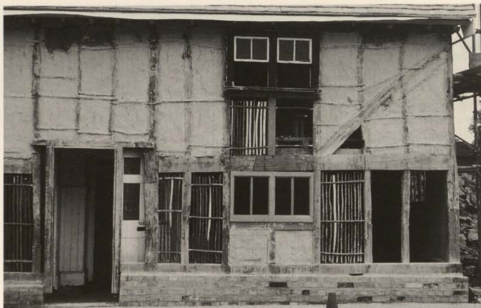
Fig. 2. Repairs using Traditional Materials. – The owner of this cottage wanted to use traditional materials to repair it. New materials can sometimes have a role in repairs, but the advantage of traditional ones is that they have been tested over hundreds of years.
