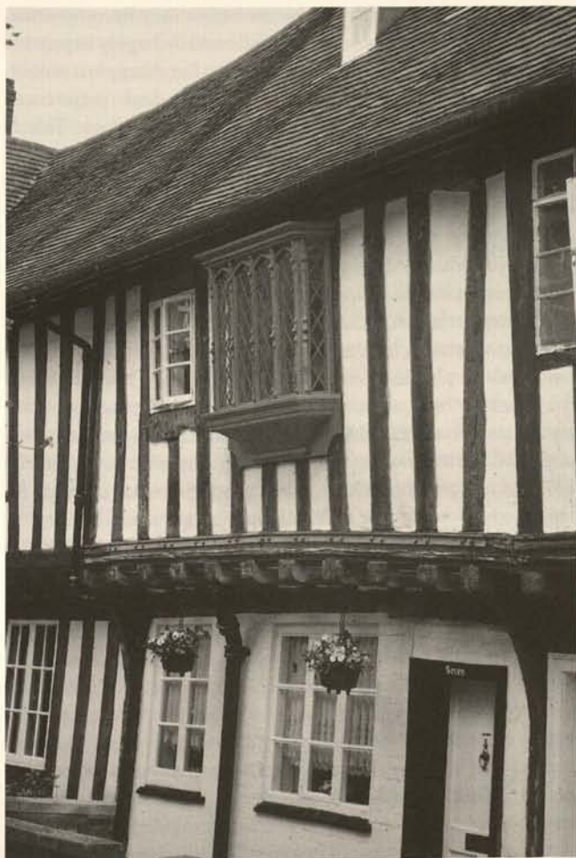
Fig. 1. Vicars Close, Lichfield. – The SPAB objects to the restoration of long vanished features, like this oriel window for which there was only the most limited archaeological evidence.
