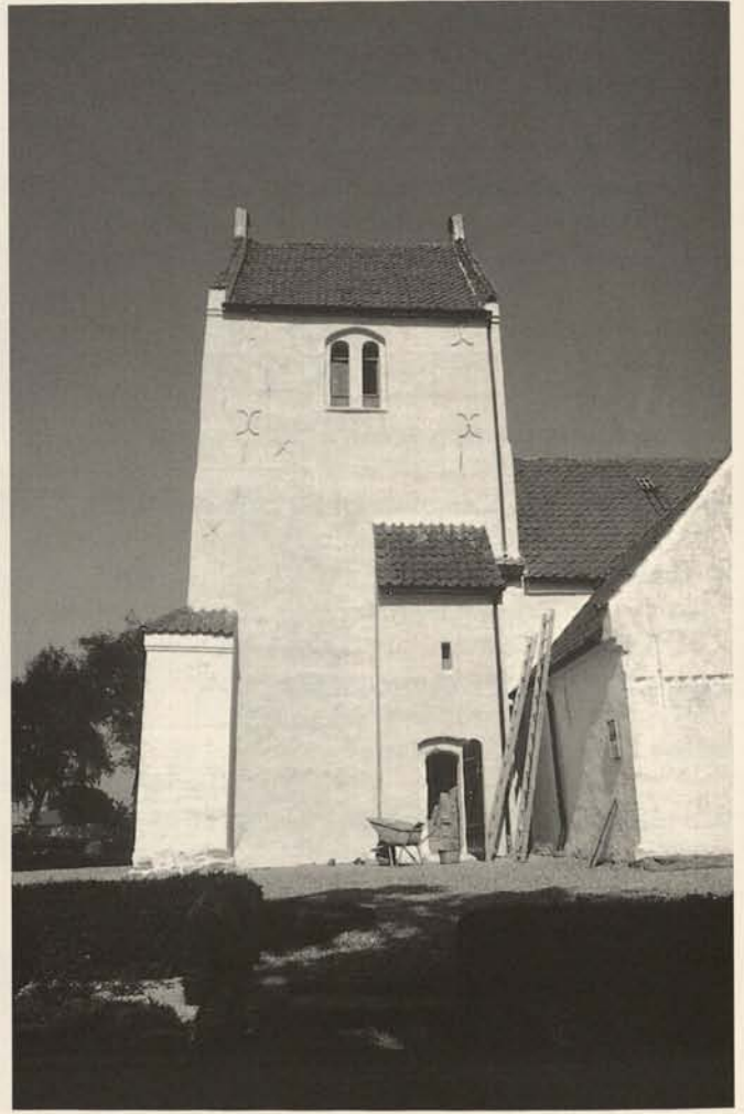
Fig. 6. Vallekilde Church (Zealand). After treatment in 1992 with a rendering made of slaked lime and aggregates up to 2,2 mm (1:2,5 volume). The church was limewashed the following year.
