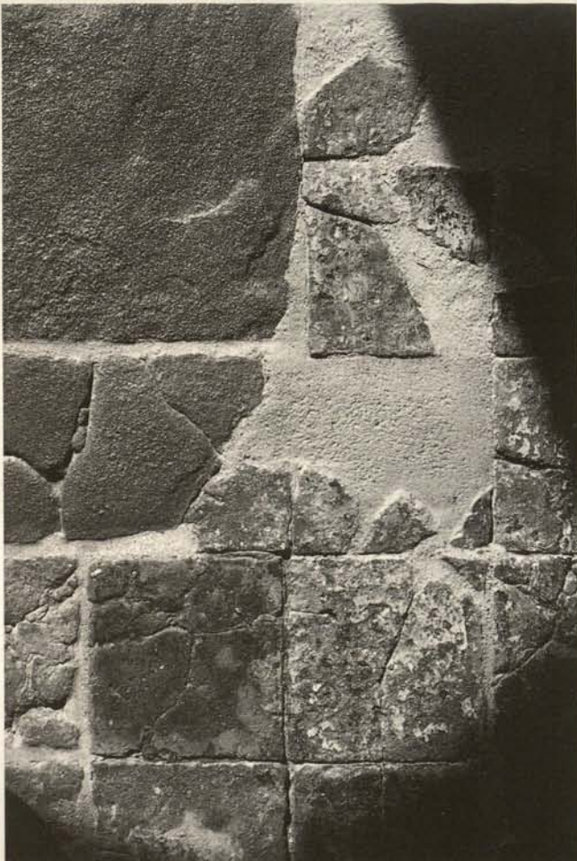
Fig. 13. Fourth case study: Acton Court. Cross passage floor on completion of lime repairs. Note area of contrasting mortar to indicate resiting of buried tiles.
