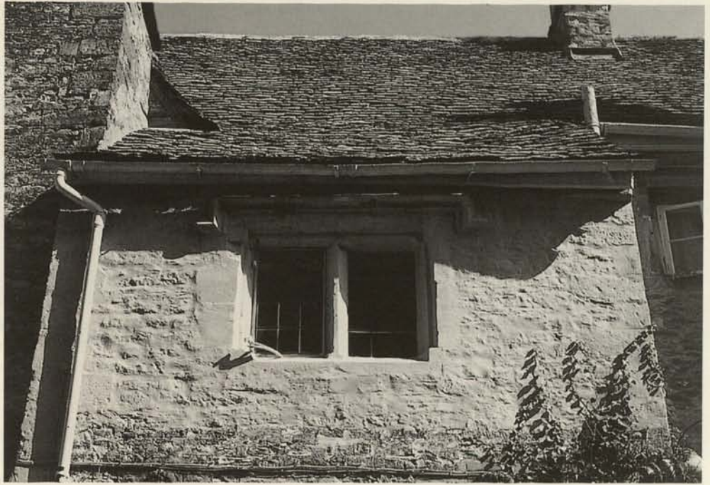
Fig. 7. Second case study: Woolgatherers staircase. Completed lime repairs to mortar joints and stones, and five coats of limewash.
