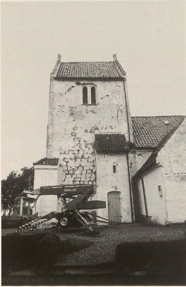
Fig. 5. Vallekilde Church (Zealand). The tower after cleaning in 1991. The lower part is made of granite boulders and the rest partly of hard-burnt bricks. In those areas, a cement slurry was preserved.
