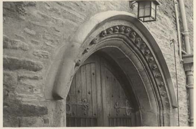
Fig. 10. Third case study: Broadfield Court. The completed lime repairs. Note the limewashed stones of the hoodmould, and repointed rubblework.
