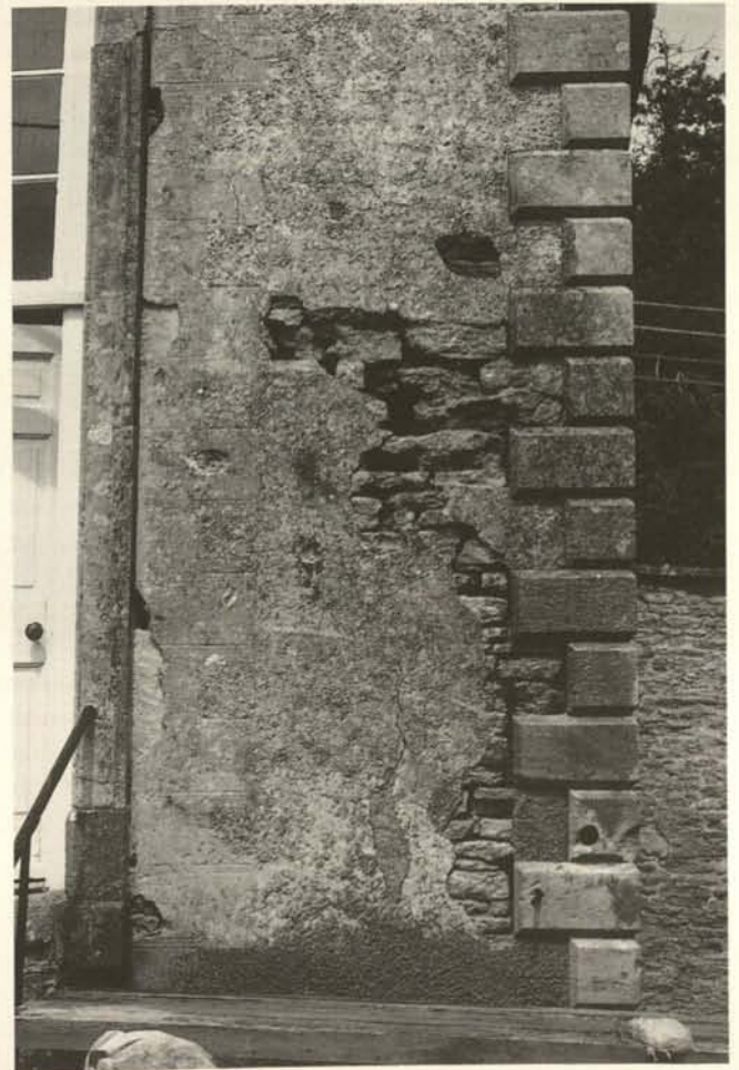
Fig. 1. First case study: Church House Gazebo. Preparation for lime mortar consolidation and lime roughcast render. Loose material was associated with settlement in the structure.
