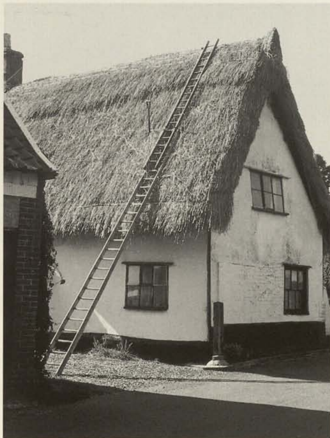
Fig. 10. Britain's buildings vary greatly from one area to another because of the changes in local building materials. It is essential that repairs recognise this, for example, in rethatching buildings with combed wheat reed or long straw, where they are traditional, rather than water reed which has a quite different appearance.
