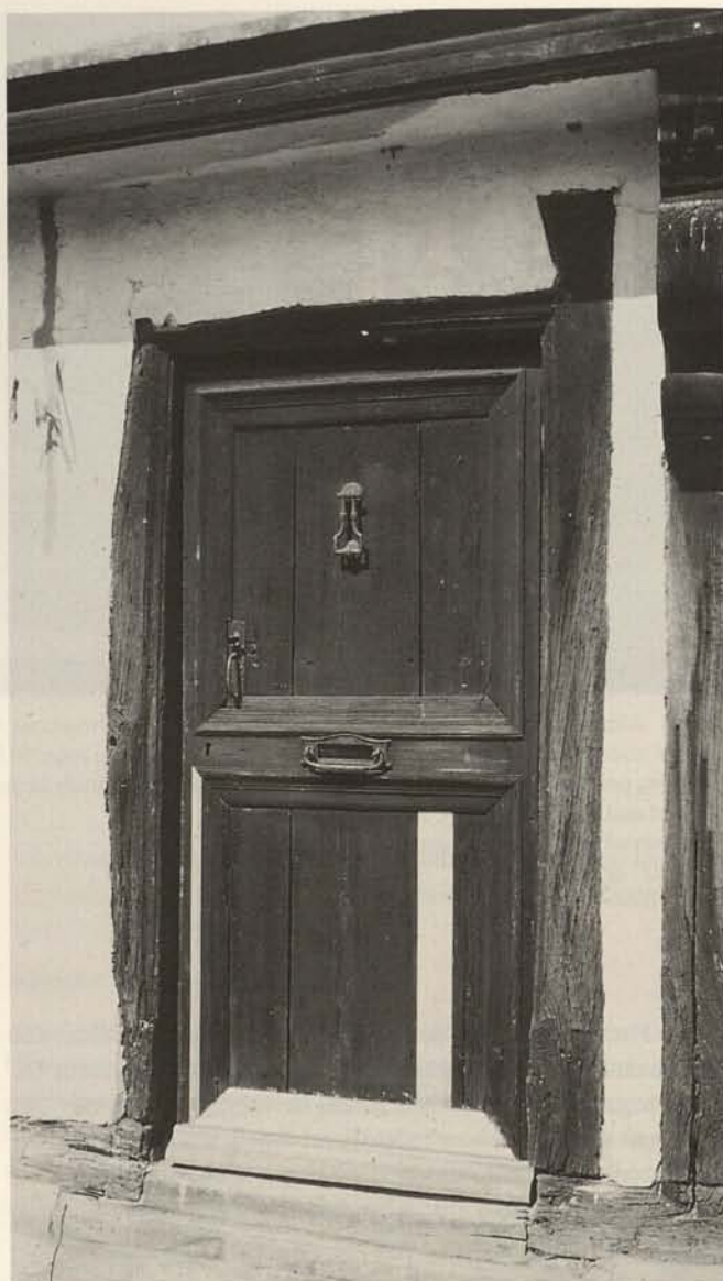
Fig. 8. Repaired Door. – A simple carpentry repair has allowed this historic door to remain in regular use, which is far preferable to its replacement with a new copy.
