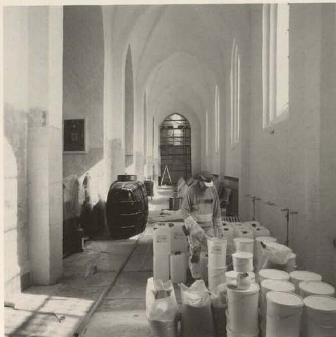
Fig. 2. Lime putty, quartz sand and limewater delivered ready for lime-washing the cathedral in Århus.
