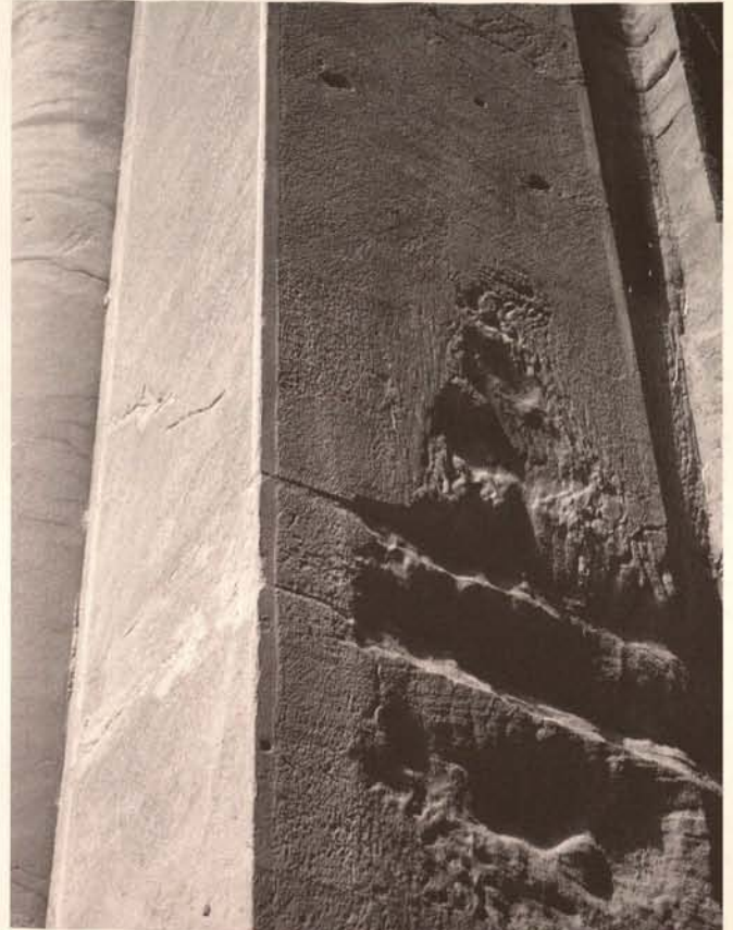
Fig. 14. Alveoles in a pillar carefully dressed with a flat and pointed chisel
