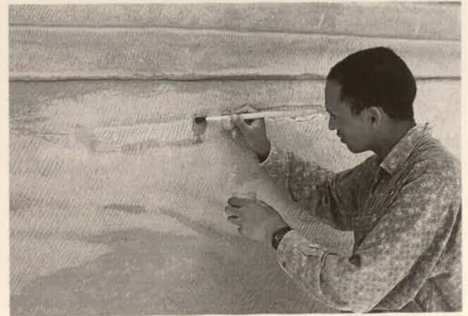
Fig. 10. Application of suspension retouching the filling
