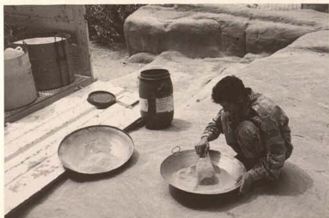
Fig. 7. Mixing in front of the scaffold
