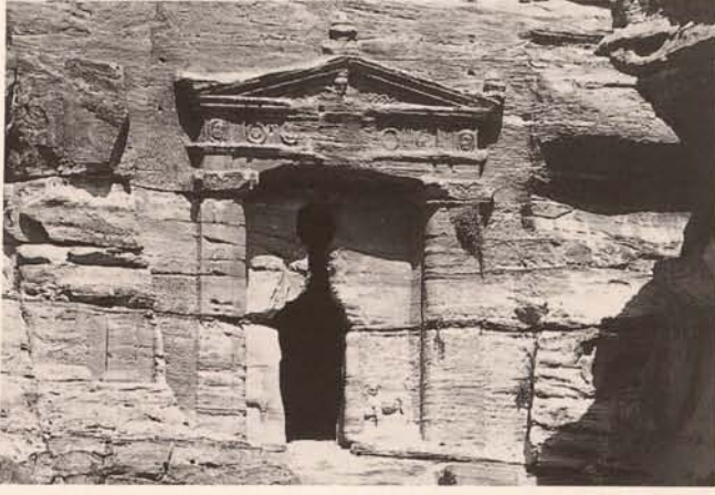
Abb. 4. Löwengrab, Riß an der Trennlage zweier Gesteinsschichten Fig. 4. Lions Tomb, crack following the line between two lithological layers
