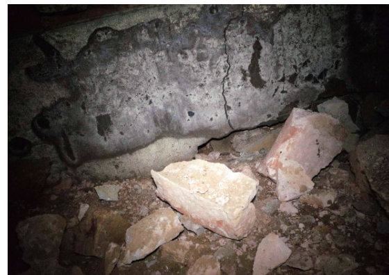
Photos 3.7.2.1 The Idera Kofun: Fissure in the mound and damaged stone chamber (courtesy of Kashima Town Board of Education).
