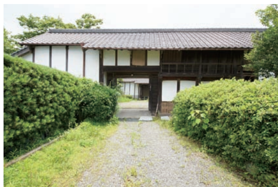
Photo 3.1.5.4 The Saionji gate house “ Nagayamon ”
