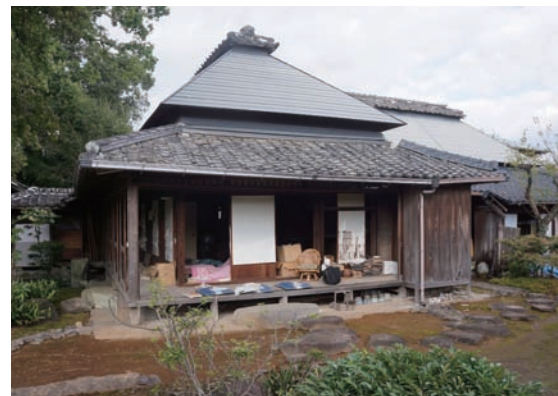
Photo 3.1.10.2 The Kimura family home: Overall appearance (from the southwest side).
