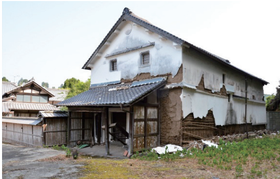
Photo 3.1.2.9 The storehouse of the Yano family home ( Hontaku )
