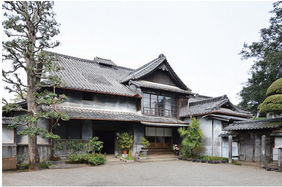
Photo 3.1.1.1 The main building (before the earthquakes)
