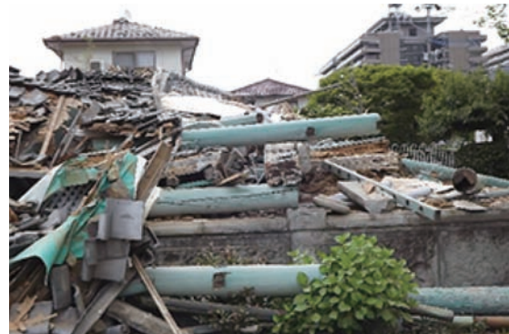
Photo 3.1.6.5 The building was completely destroyed in the main-shock earthquake (1).
