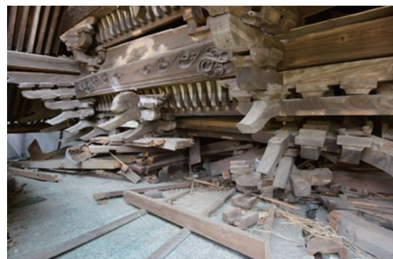
Photo 3.1.5.2 The decorated structural element which joins columns and the beams of a roof. (Sculpture of Horeki Era.)
