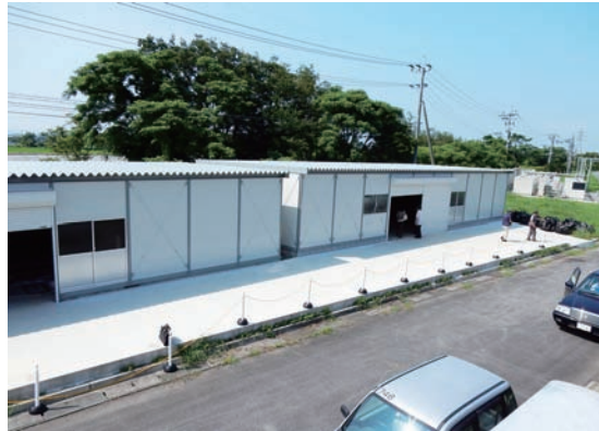
Photo 3.1.6.8 The three warehouses to which the dismantled Janes House's building materials had been transported and are being preserved.
