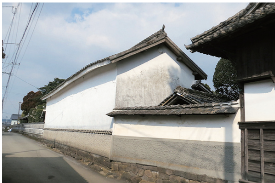
Photo 3.1.1.5 The stable (before the earthquakes)
