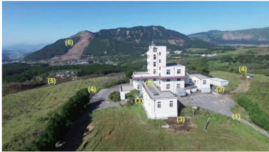
Photo 3.3.2.1 This is an aerial photograph taken of the Aso Volcanological Laboratory and its surrounding area on October 24, 2016. In the far distance can be seen Mount Unzen on the Shimabara Peninsula. Below are the explanations of (1) to (6) in the photograph.
