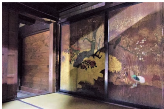
Photo 3.1.7.4 Additional earthquake-resistant walls (left side of the wooden door).
