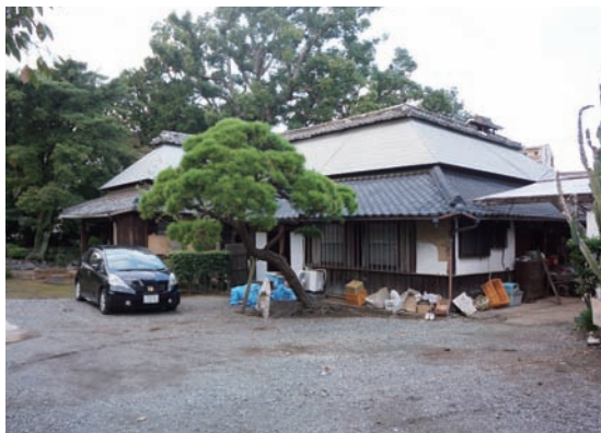
Photo 3.1.10.1 The Kimura family home: Overall appearance (from the southeast side).
