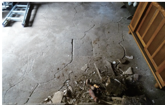
Photo 3.1.2.8 The fissure in the earthen floor of the main building of the Yano family home ( Hontaku )
