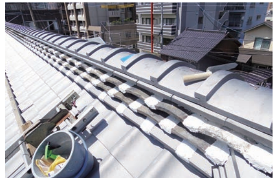
Photo 3.1.7.6 Restoration of the large building using the original tiles (main building).
