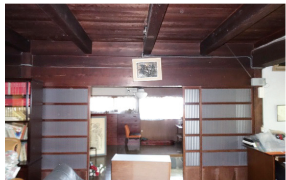
Photo 3.1.2.12 A sashigamoi (heavy head jamb) of the Yano family home ( Shintaku )
