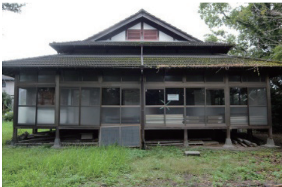
Photo 3.4.2.9 The Kawashiri Public Assembly Hall
