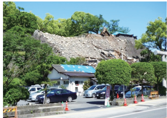
Photo 3.7.1.8 The Higashi Juhachiken Turret after the damage
