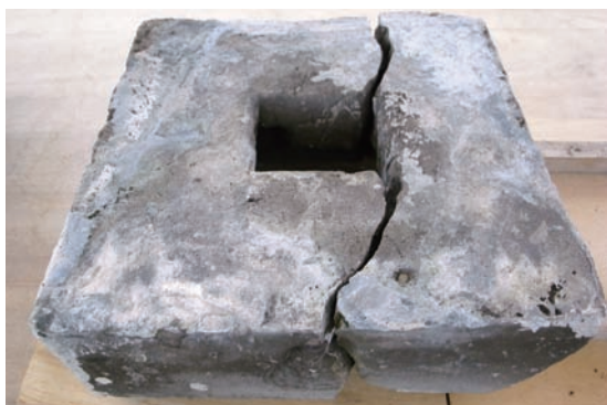
Photo 3.6.2.4 The damaged fifth story of the pagoda
