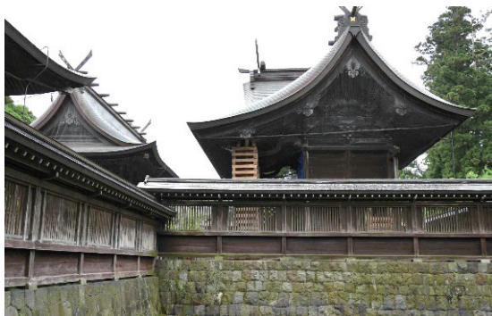
Photo 3.1.3.3 The Worship Hall of the Aso-jinja Shrine was damaged.
