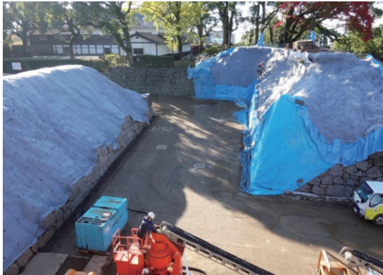
Photo 3.7.1.4 Emergency measures taken at the Suki-yamaru Gate site (from the West)
