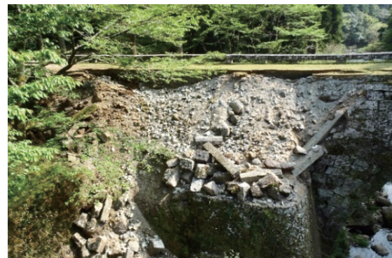
Photo 3.6.1.4 The stone wall on the upstream side collapsed at the Yasemegane Bridge (Photo by Mifune town)
