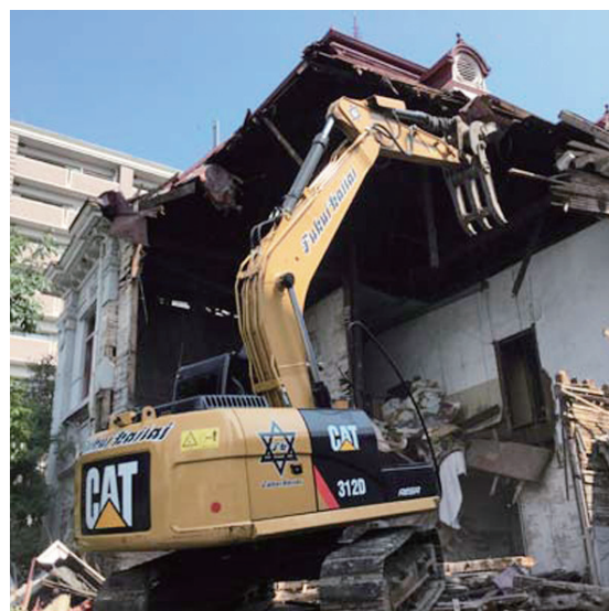
Photo 3.4.1.4 A townscape-formation building being dismantled (July 2017).
