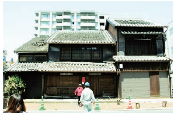
Photo 3.1.8.2 Dismantling work by volunteers for its relocation.
