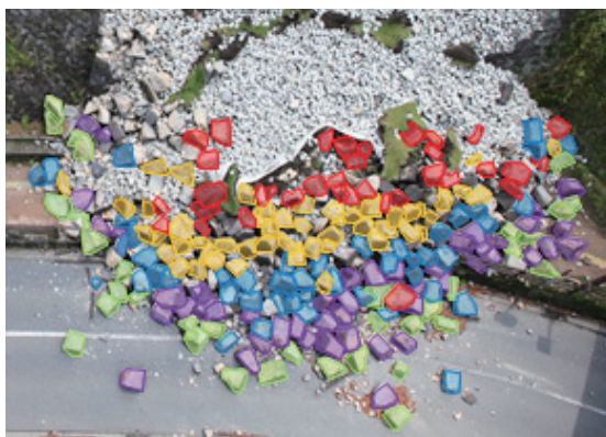
Figure 3.7.1.10 The collapsed Miyauchi dry stone wall
