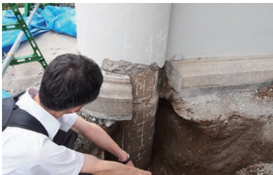
Photo 3.3.1.5 Honmyo-ji Nio-mon: the state of the ground around the column base.
