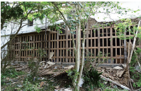
Photo 3.1.2.10 The storehouse of the Yano family home ( Hontaku )
