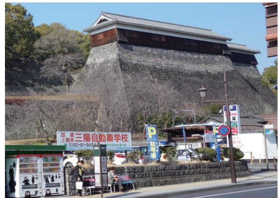
Photo 3.7.1.7 The Higashi Juhachiken Turret before the damage
