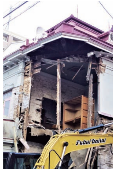
Photo 3.1.9.3 During the dismantling.
