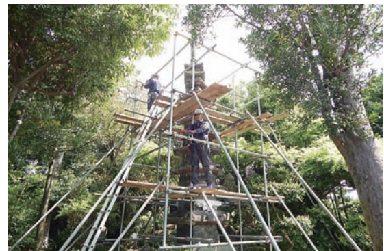
Photo 3.6.2.3 The dismantling of the upper part (April 19th, 2016)
