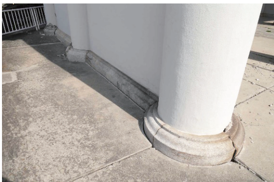
Photo 3.3.1.3 Honmyo-ji Nio-mon: column bases and the surrounding area.
