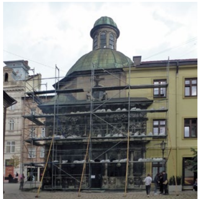
Fig. 5 Construction for the protection of the monument to A. Mickiewicz. Fig. 6 Construction for the protection of the memorial column of St. John. Fig. 7 The first stage of protecting the stone sculptures of the Campian Chapel. Fig. 8 The process of installing protection on the facade of the Boim Chapel
