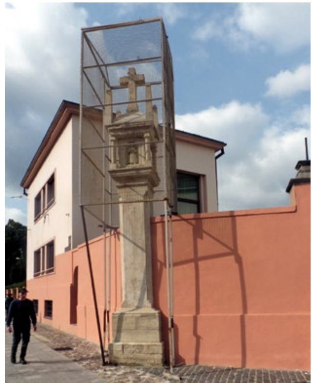
Fig. 1 Structure to protect the stone sculpture of the Greek god Neptune in Rynok Square. Fig. 2 The first stage of protecting stone sculptures on the fence of the cathedral. Fig. 3 The cage-like structure is installed to protect the stone sculpture on the fence of the cathedral. Fig. 4 Protection of the Sykst Chapel
