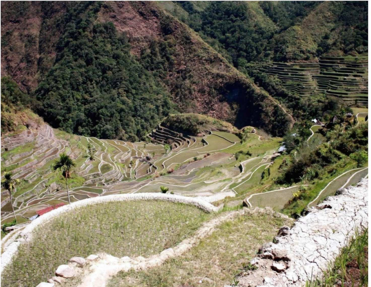
Fig. 25. Terrace walls are dried and cracked during drought. (Source: SitMo 2017)
