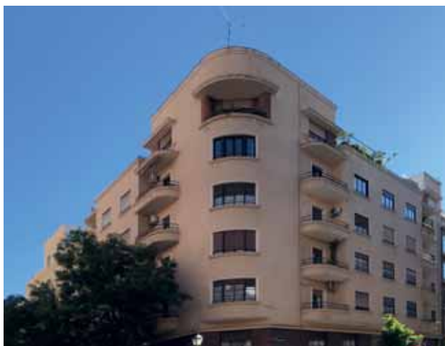
Fig. 4 Residential building at Fernández de los Ríos 53, by Luis Gutiérrez Soto, 1930
