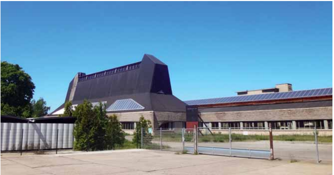
Fig. 9 Dyeing and production workshops, power station (in the background) of the Hat Factory in Luckenwalde, 2017
