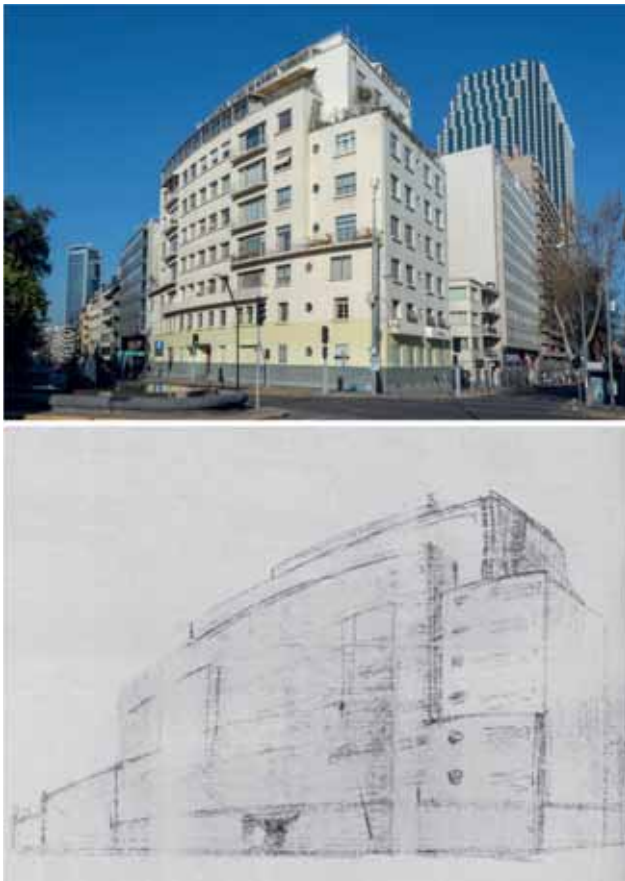
Fig. 9 Santiago de Chile, Edificio Santa Lucia, Sergio Larraín, sketch of the facade and situation today
