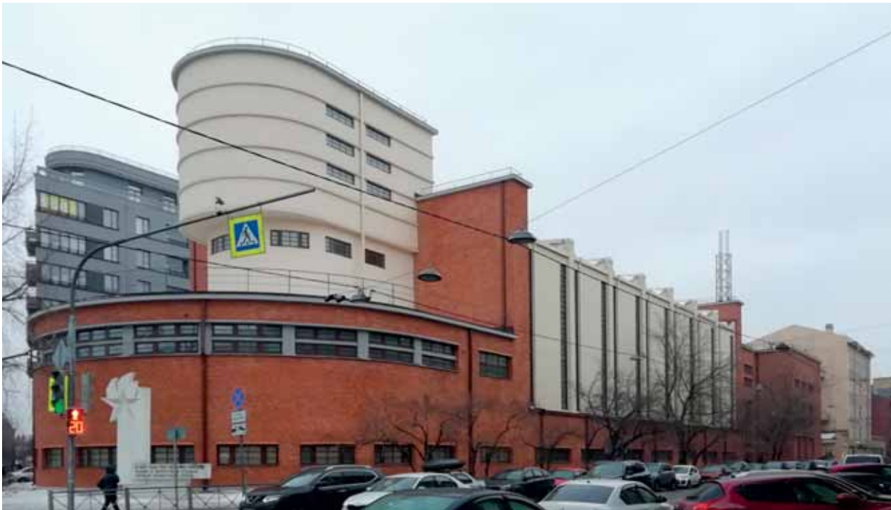
Fig. 7 Power station of the Red Banner factory, 2022
