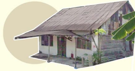
Timber structure house with masonry works and zinc roof sheets
