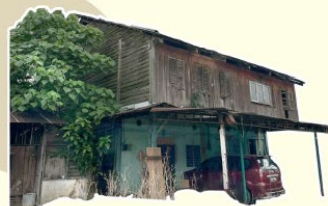
Two storey houses with masonry brick and timber
