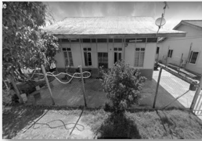
Single-storey wooden house for a Hakkan household
