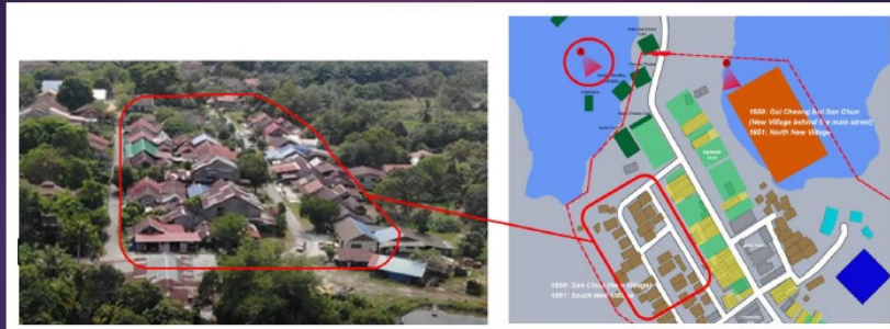
Drone view A: These rows of village house initially called South New Village. Some houses on the left row were built on vacant lots that originally were commercial lot. Both Papan Heritage Gallery and Malaysia New Village History Gallery were located at this row. The middle and right rows have 4 double-storey wooden shophouses built before Briggs Resettlement Plan and some of the most authentic and best-preserved New Village houses, together it formed the best combination that inspired the Papan Conservation Group to make these rows of house as "Live Museum of New Village" in the State.
