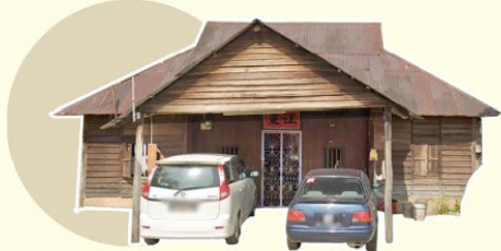
Full timber structure house with gable roof, similar to Malay kampung house
