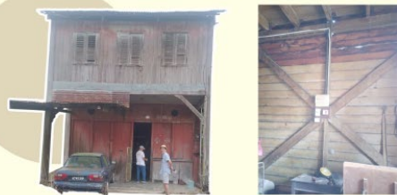
Two storey full timber house with timber trusses and structural wall bracing
