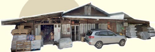
Full timber house metal sheet roof
