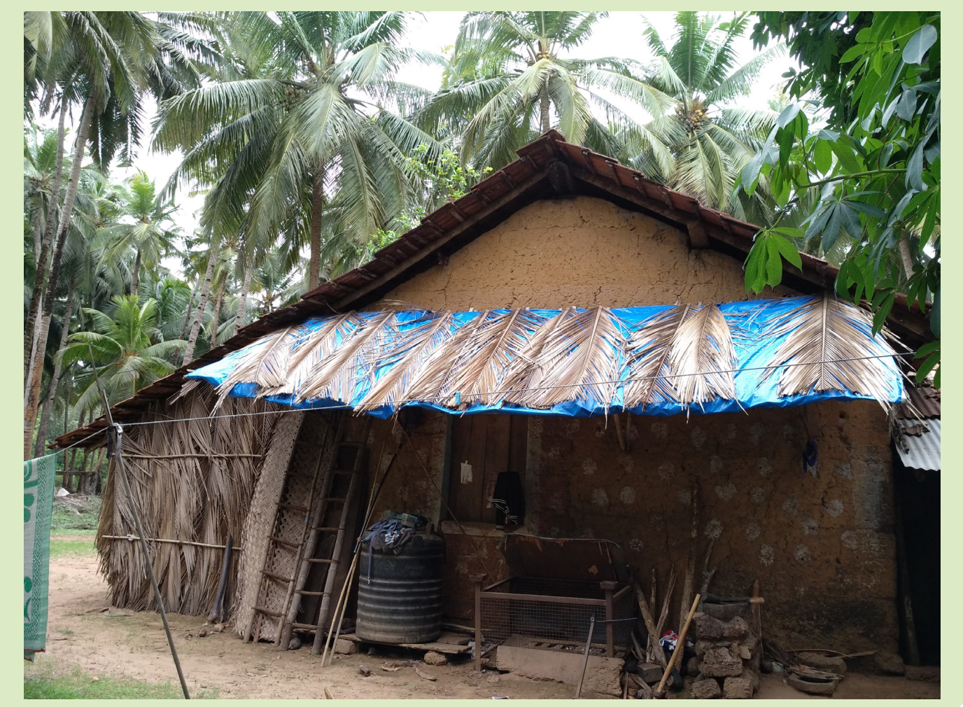
Large overhangs built with local materials. Goa (2019) [Photo credit: Chenelle Rodrigues]
