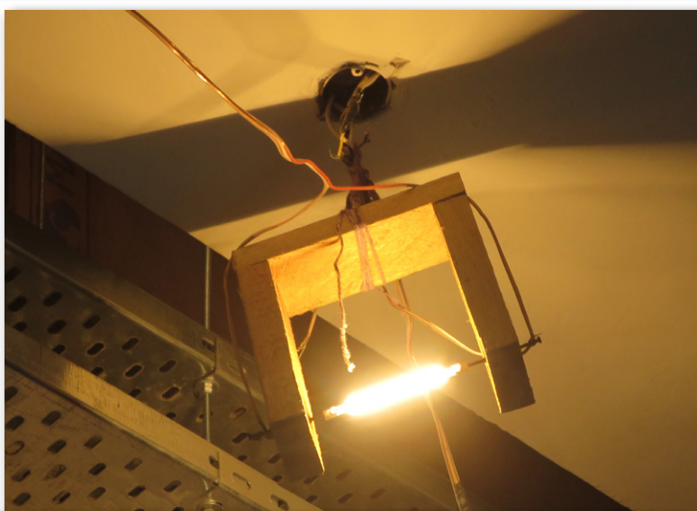
Figure 44. Makeshift lighting, heating and other equipment may create ignition sources throughout a site/structure.
