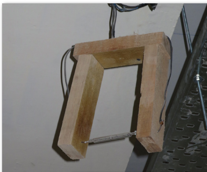
Figure 44. Makeshift lighting, heating and other equipment may create ignition sources throughout a site/structure.
