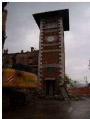
Fig. 6: Demolition of the Sušak Railway Station (photo by Nana Palinić)
