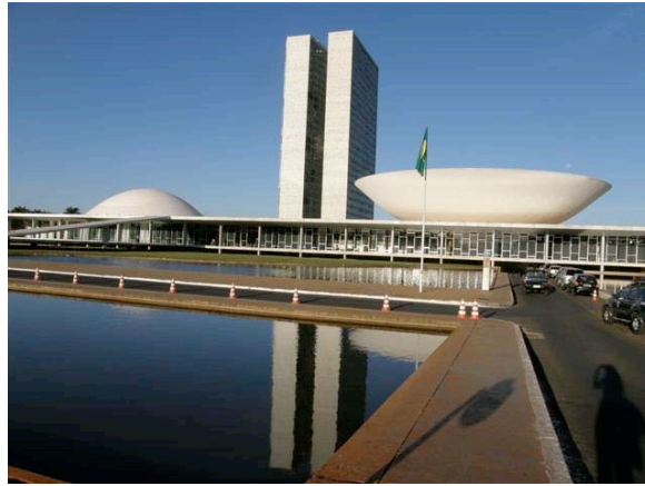
Figure 7. Brasília, Brazil's capital since 1960 is an example of the application of the principles of the Athens Charter.
