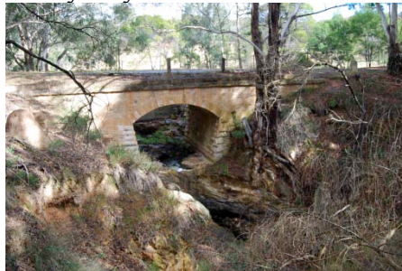
Fig.2 Towrang Road Bridge
