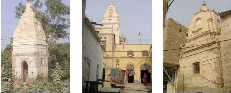
Figure 5. The surviving examples of the conical temple structures.
