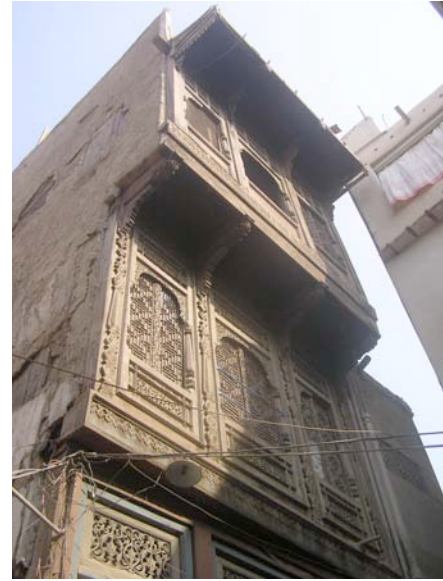
Figure 7. Façade of a traditional residence completely adorned by fine details including screens, carvings and brackets made with timber.
