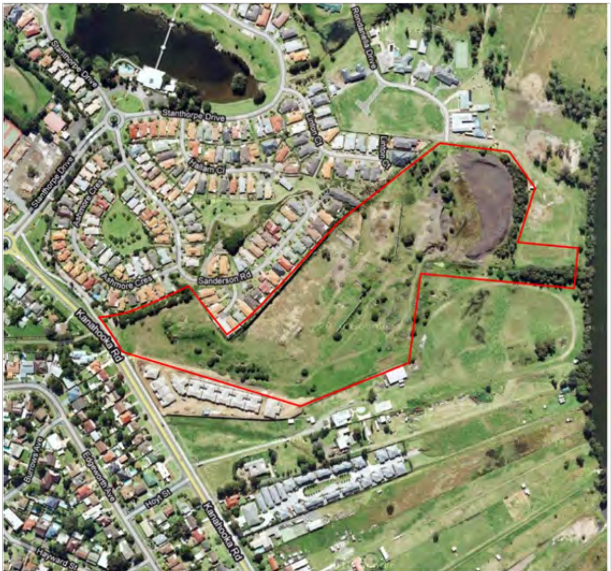
Figure 2. Aerial photograph of the Brooks Terrace development site which occupies the eastern portion of the former Dapto smelter site. The approximate boundary of the site is outlined in red. During the 1990s the land to the northwest was redeveloped for the residential purposes. (Google Map, 2011)
